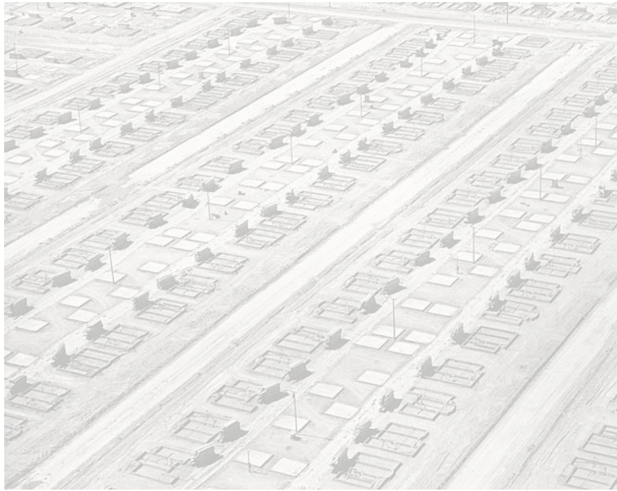
Fig. 57 William Garnett, Foundations and Slabs, Lakewood, CA , 1950. Silver print. 7 7/16 x 9 3/8 in.
