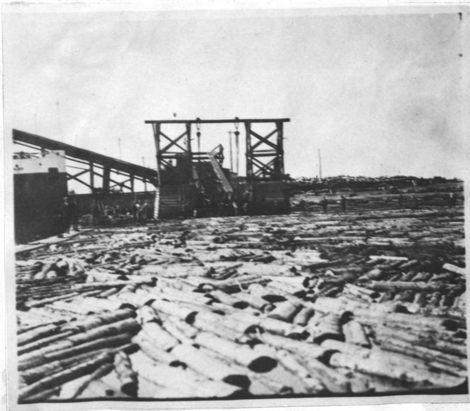
Fig. 17. Wood floating in dredged log pond ready for transfer by jackladder to main trestle for loading.
