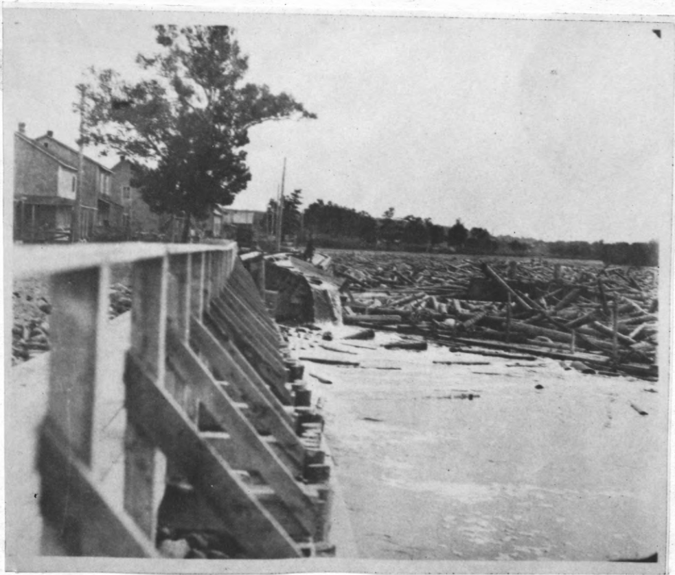
Fig. 13. Outlet of flume which discharges wood into pond. (Note log-jam in river at right.)
