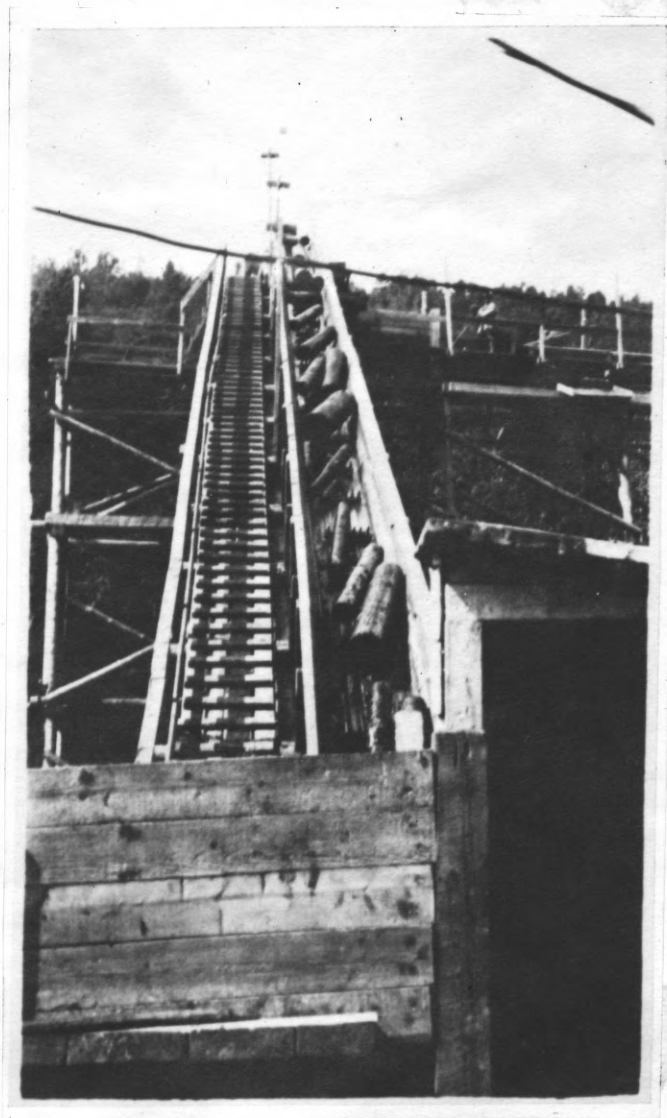
Fig. 18. Jackladder used in transferring wood from pond to main trestle.
