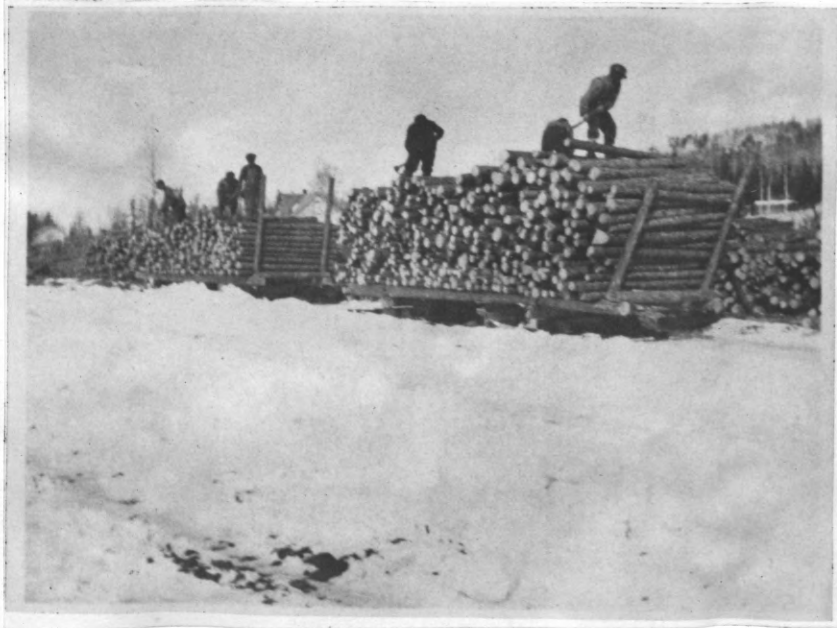
Fig. 6. Unloading pulpwood from sleighs to river.
