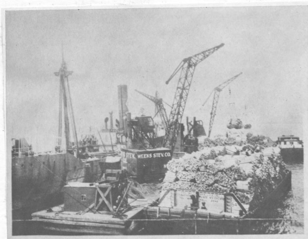
(Fig. 17) Loading bundles of pulpwood on ship from a barge which has been towed alongside the ship.
