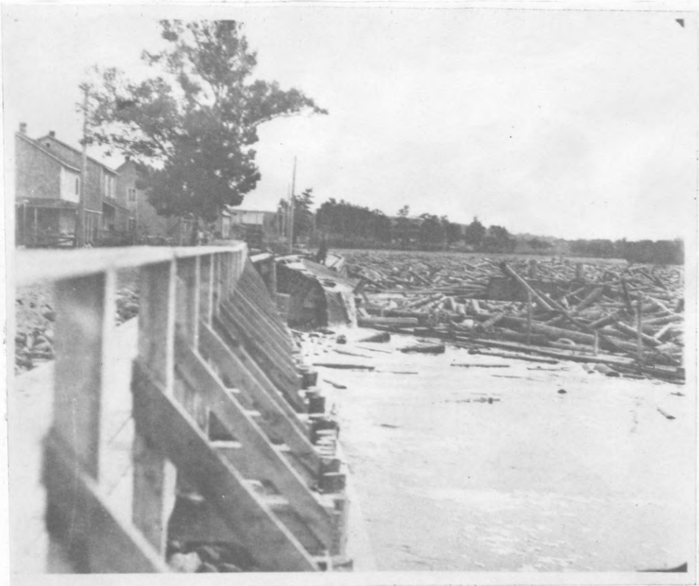
(Fig. 10) Lower end of flume emptying into storage pond.
