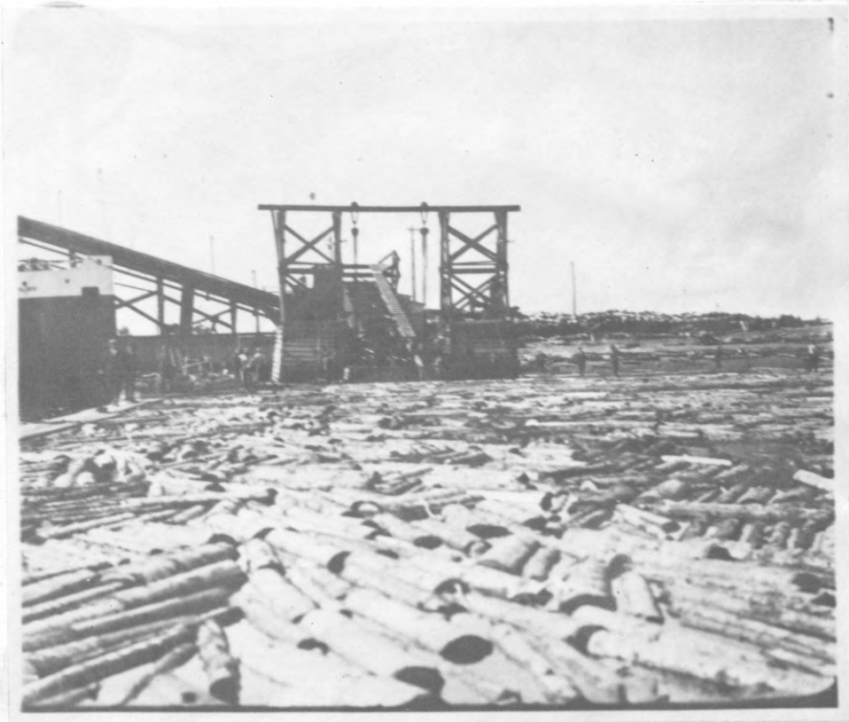
(Fig. 14) Pulpwood in storage boom at loading deck, showing part of loading conveyor.
