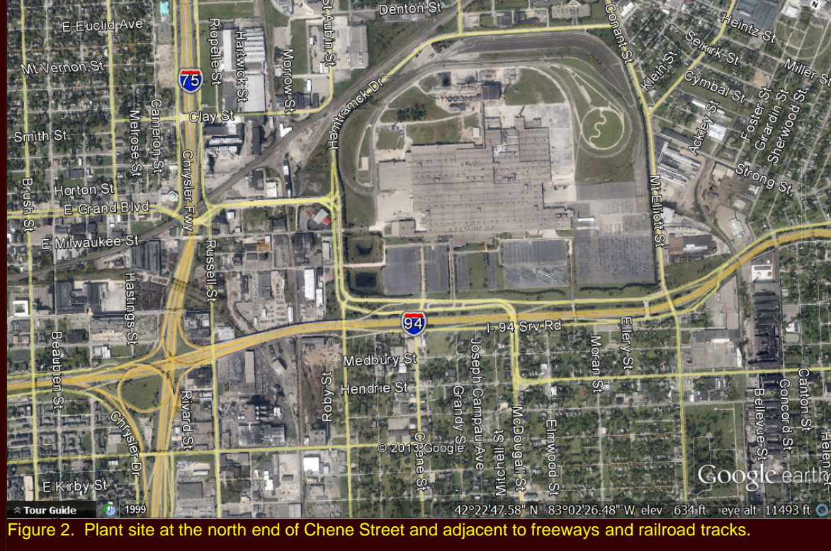
Figure 2. Plant site at the north end of Chene Street and adjacent to freeways and railroad tracks.
