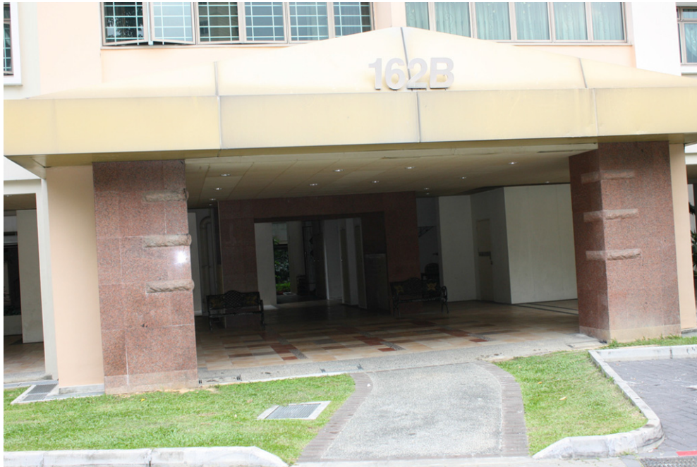
Figure 2 Void Deck, Senkang New Town (photo by the author, 2010)
