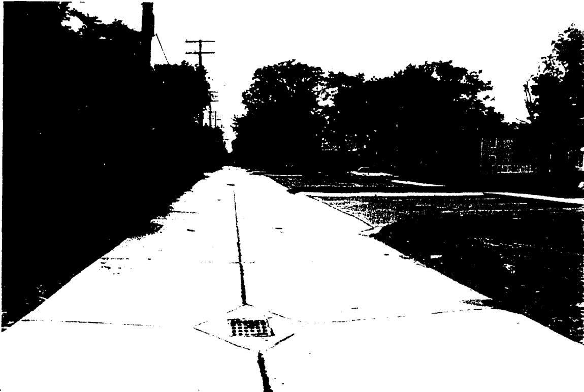
Figures 4.9 Before and After Photographs of Renovated Alley Between Field Street and East Grand Boulevard
