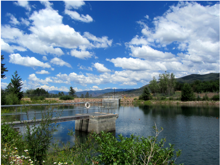
Figure 1: Water storage reservoir at the City of Aspen Water Department.
