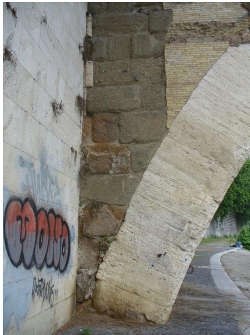
Figure 35: Pons Fabricius. Both gray lapis Gabinus and reddish tufo lionato are visible in the facing. The arch is travertine.
