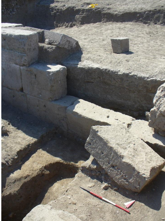
Figure 48: Mid-Republican retaining wall at Gabii composed of lapis Gabinus.
