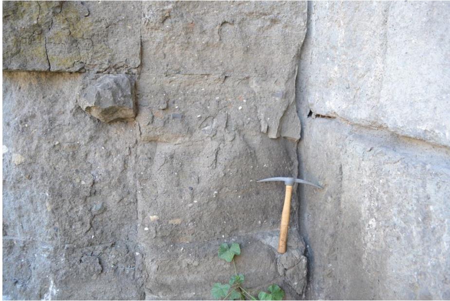
Figure 42: At left, lapis Gabinus blocks in the apses of the Forum of Augustus. At right, lapis Albanus in a later abutting wall.
