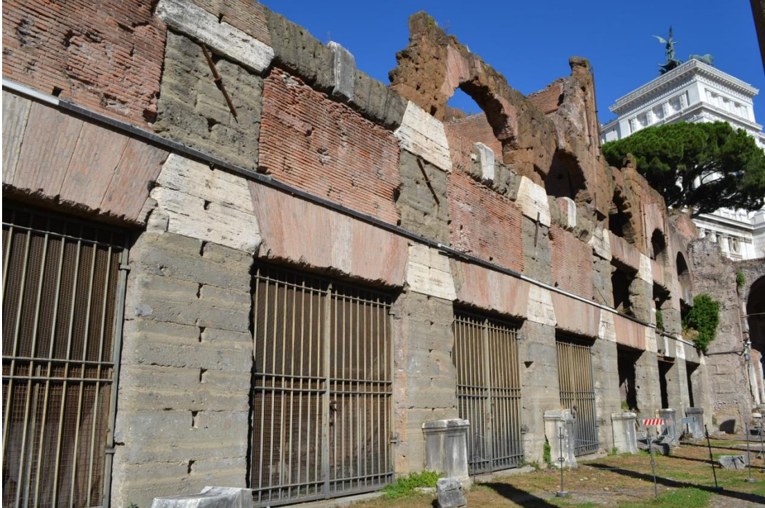
Figure 38: The tabernae in the Forum of Caesar, with lapis Gabinus piers and flat arches.
