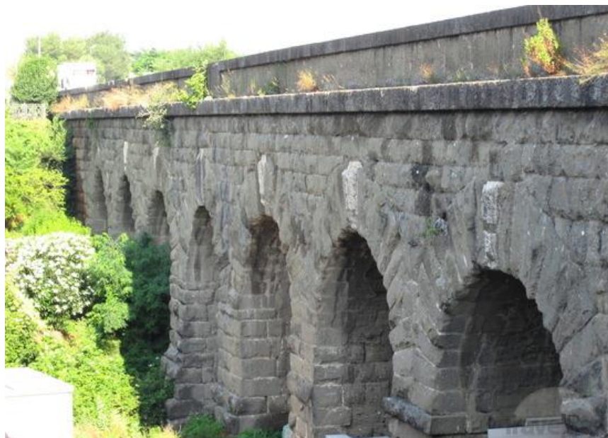
Figure 45: The Ponte di Nona, constructed largely with lapis Gabinus.
