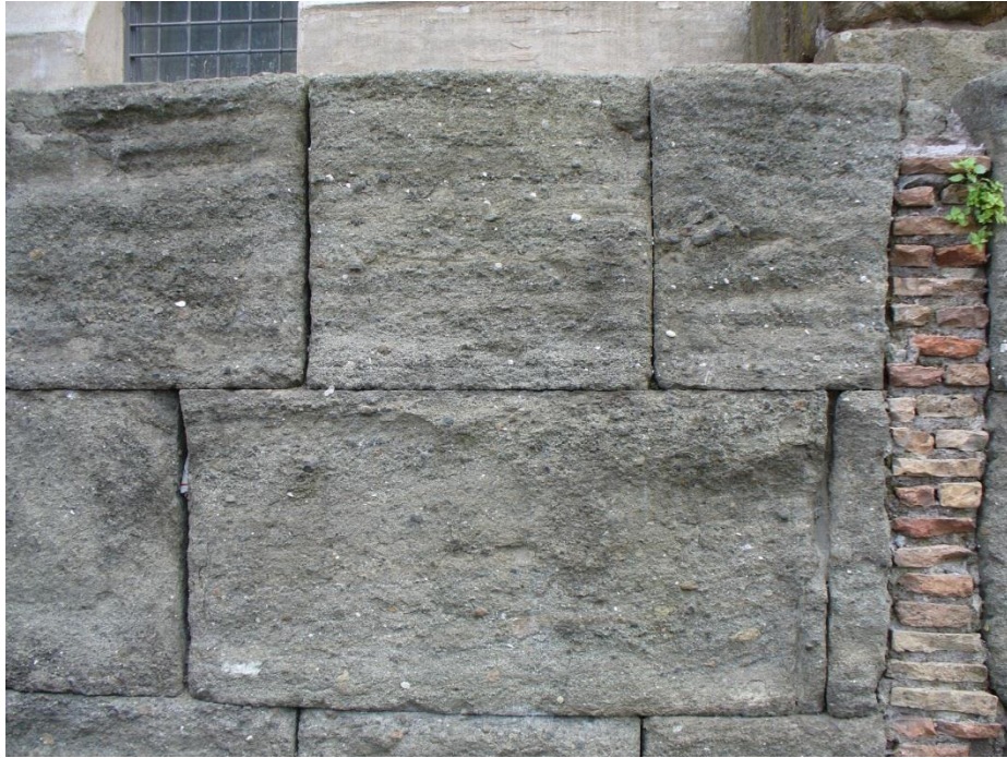
Figure 34: Lapis Gabinus in the foundations on the north side of the Tabularium
