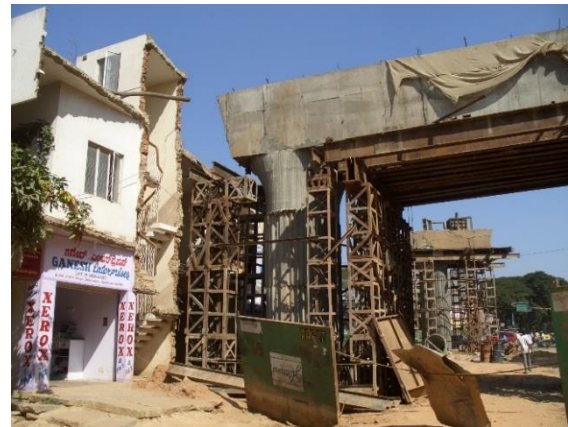
Picture 4.14. Demolished buildings to make space for Metro, CMH Road Indiranagar
