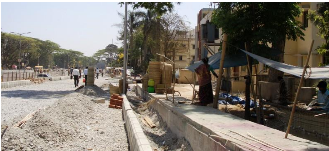
Picture 4.22. KR Road after Metro work began
