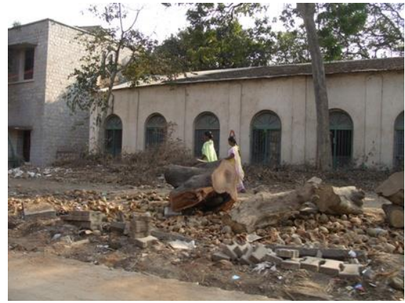
Picture 5.8. Tree felling in preparation for road widening, Sheshadripuram
