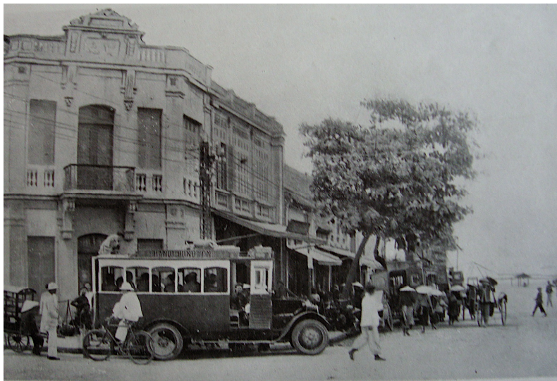
Photograph 16. Bus stop in Hà Nội, mid-late 1920s.
