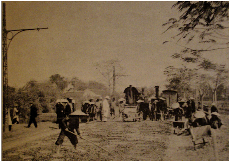
Photograph 13. Road construction, c. 1925.
