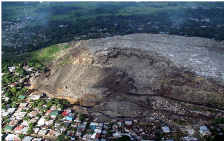
Figure 1.3 Payatas Landfill failure (Merry et al. 2005).
