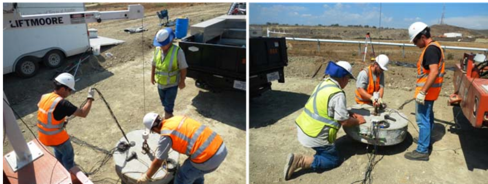
Figure 4.10 Installation of concrete footing.
