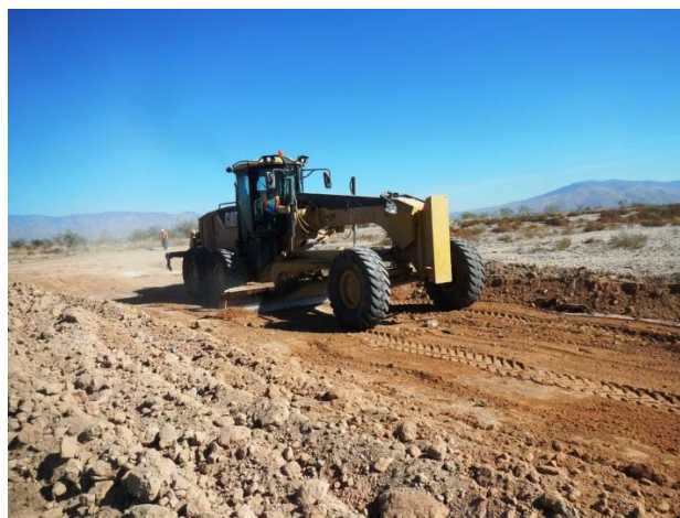
Figure 4.6 A road grader removing soil cover at Los Reales Landfill.
