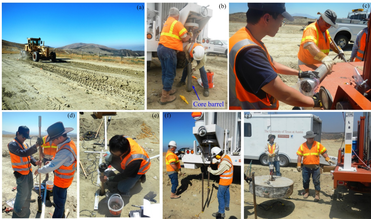
Figure 6.6 Field instrumentation and testing setup at the LCSL: (a) removing cover soil, (b) pushing core barrel, (c) removing waste from core barrel, (d) 3-D geophone installation, (e) compaction of sensor hole, (f) crosshole source rod installation, and (g) footing placement.
