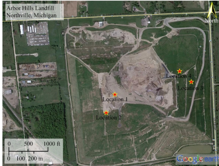
Figure 3.8 Surface wave testing locations in the Arbor Hills Landfill.
