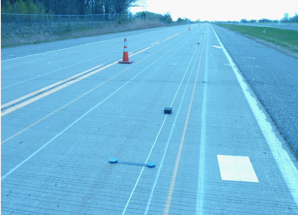
Figure A-7. Transverse tining downstream view.
