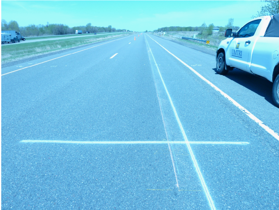
Figure A-1. Dense graded asphalt, downstream view with markings and chalk line.
