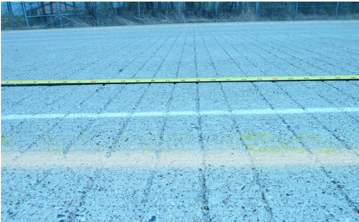
Figure A-8. Transverse tining texture.
