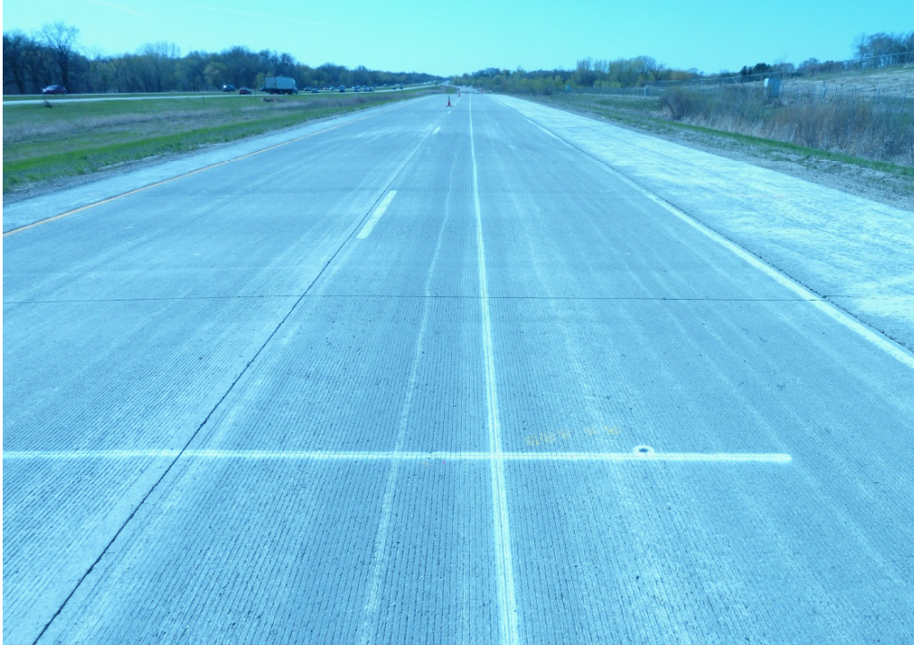
Figure A-9. Longitudinal tining downstream view.
