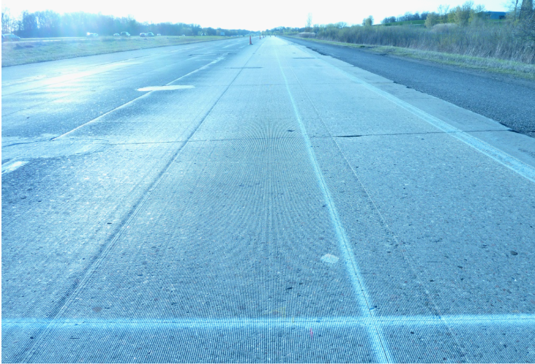
Figure A-11. Diamond grinding downstream view.
