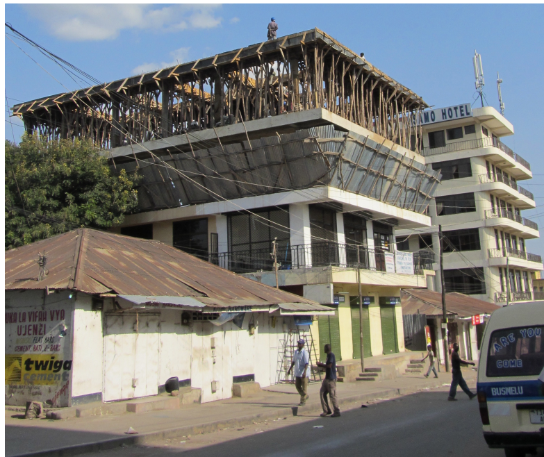
Figure 43: Incremental Formal Private Redevelopment in Mwanza
