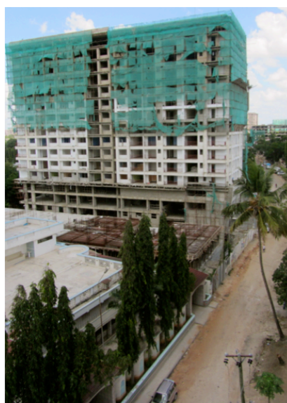
Figure 26: Road condition on Mindu Street
