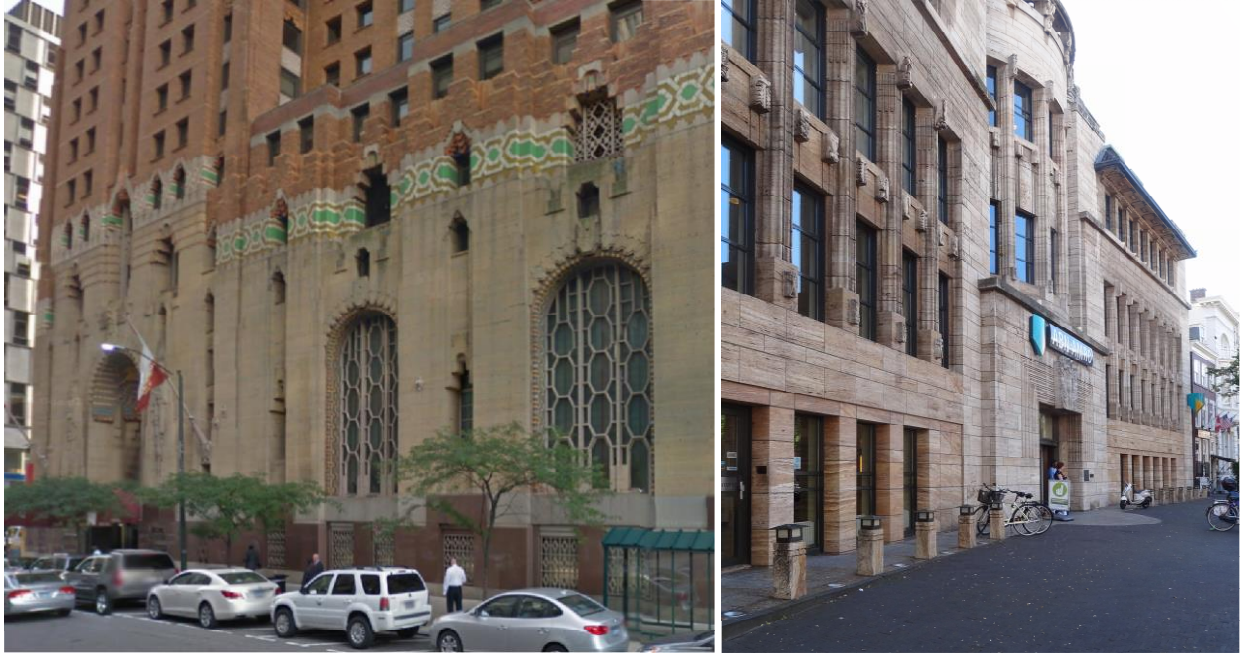
Figure 339. Guardian Bank by Smith, Hinchman & Grylls in 1929 in Detroit (left), Rotterdamse Bankvereniging designed in 1923 by H.F. Mertens in The Hague, with ground floor windows added at a later stage (right). 1301
