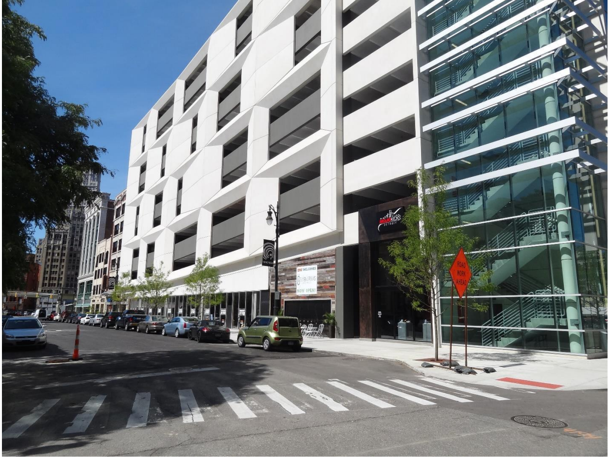
Figure 282. Z Lot parking garage above ground floor retail, with new businesses on Library Street in the background. 1165
