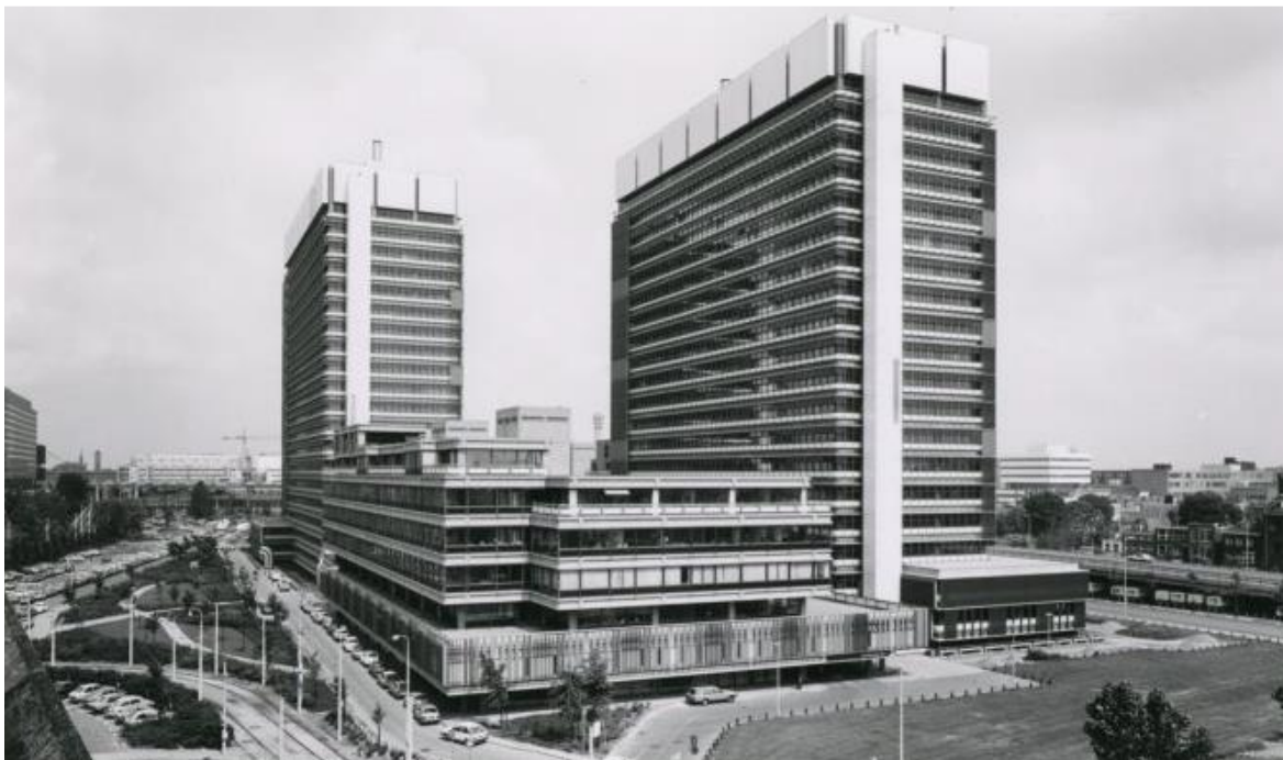
Figure 256. Ministries of Justice and Internal Affairs by Lucas and Niemeyer (1978) under construction. 1068
