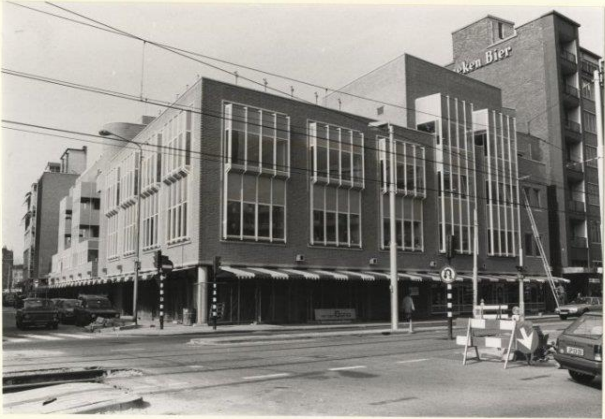
Figure 246. Markthof complex as seen from the Spui in 1983. 1044
