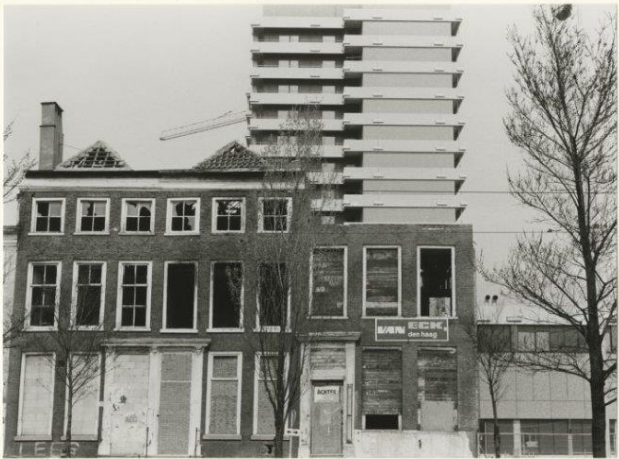
Figure 159. The new Westeinde hospital under construction behind a series of vacant buildings on the Prinsegracht. 869
