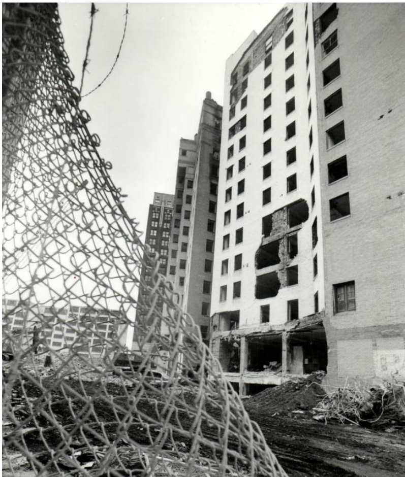
Figure 116. Demolition of the vacant Tuller Hotel in downtown Detroit, 1991. 683
