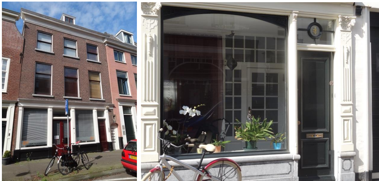
Figure 28. Many former retail stores in The Hague now serve as offices (left) or dwellings (right) by decreasing its visual permeability. 297
