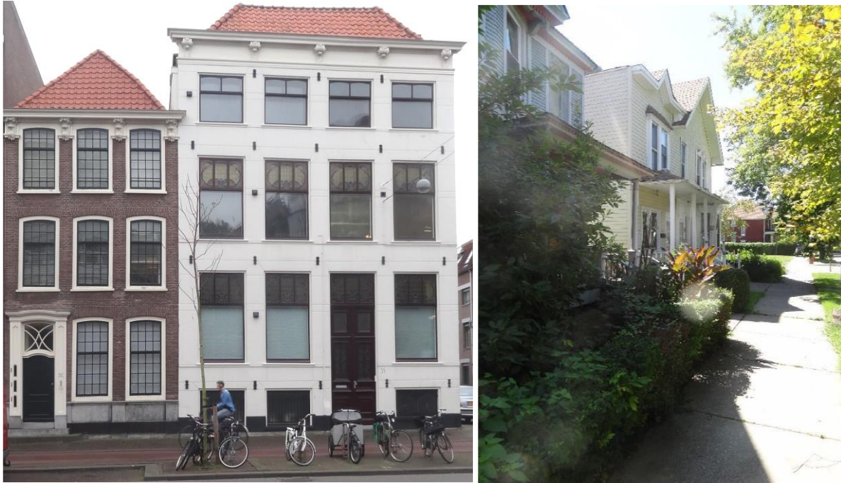
Figure 335. Transition zones between dwellings and public space, either via stoops and height as on the Amsterdamse Veerkade in The Hague (left), or by distance and territorial markers such as vegetation and porches as on Abbott Street in Detroit (right). 1297
