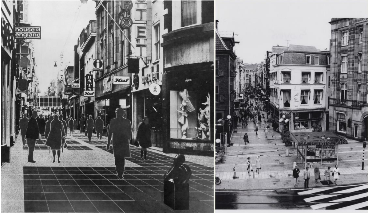
Figure 156. Photo montage of the intersection Venestraat-Spuistraat-Wagenstraat-Vlamingstraat (left), finalized 'Palace Promenade' with kiosk around 1965 (right). 847
