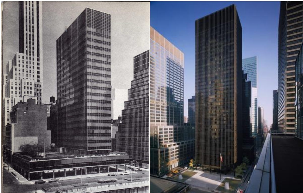
Figure 25. Left: The 1952 Lever Building constructed on top of an elevated podium. Right: The 1958 Seagram building is set back, leaving room for Seagram Plaza. 223
