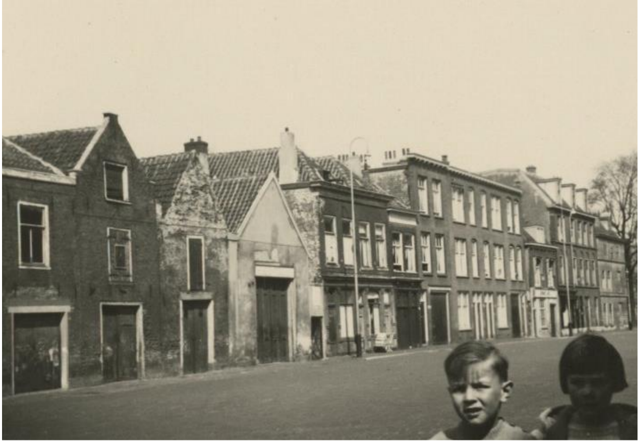
Figure 254. Deterioration and vacancy along the filled Schedeldoekshaven around 1950. 1062
