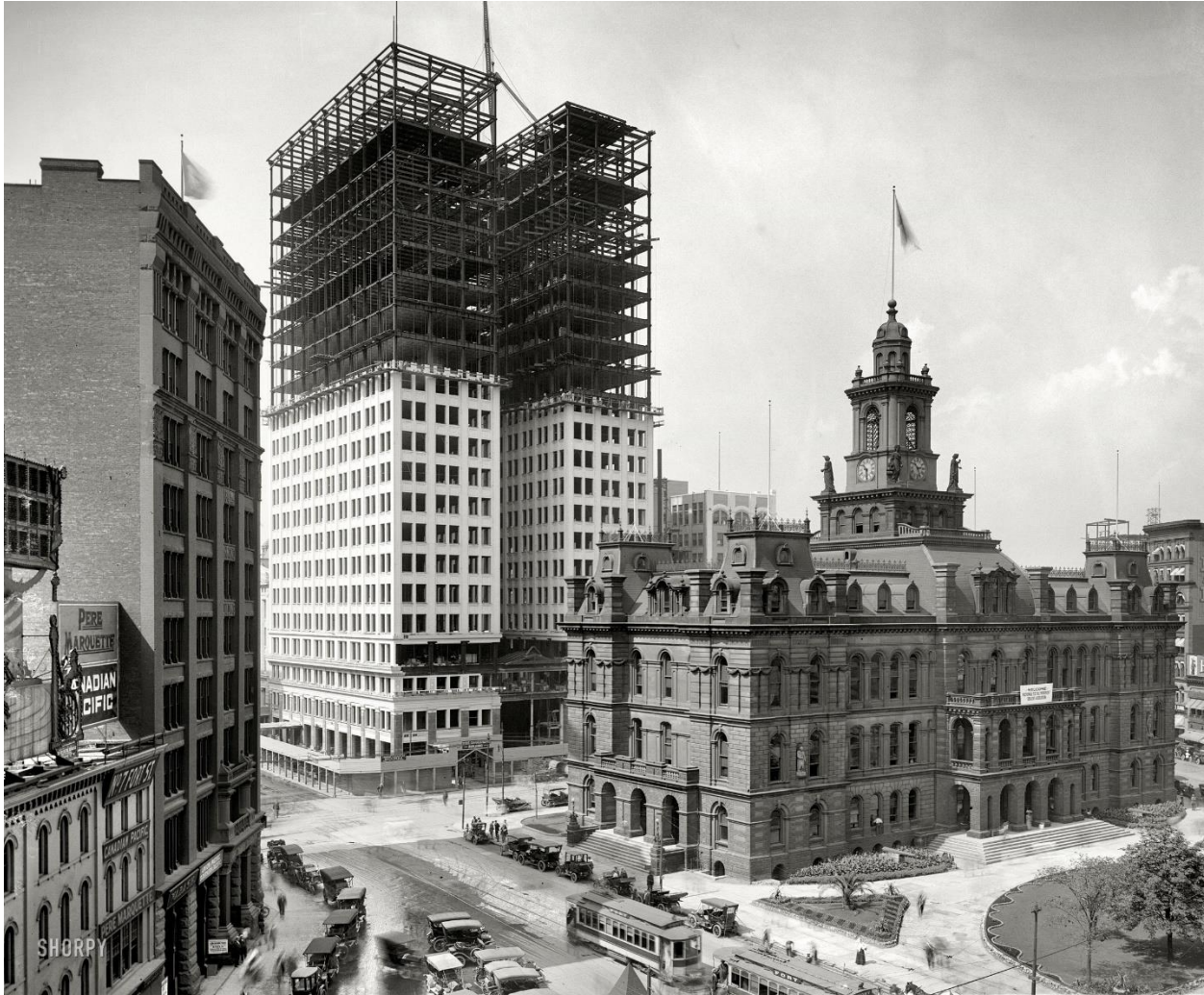
Figure 63. Dime Building under construction behind old City Hall in 1912. 388
