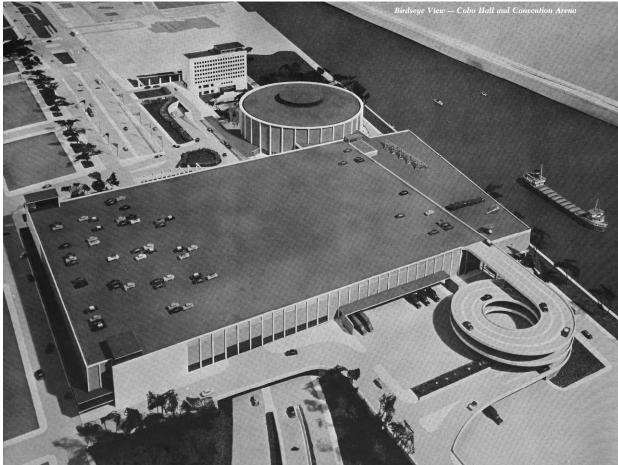
Figure 97. Rendering depicting Cobo Hall with John C. Lodge Expressway in foreground, parking ramp to roof deck to the right and convention arena in the background. Note that no surrounding buildings other than the Modern Veterans’ Memorial Hall were included in this rendering, most likely by architects Giffels and Rosetti. 551
