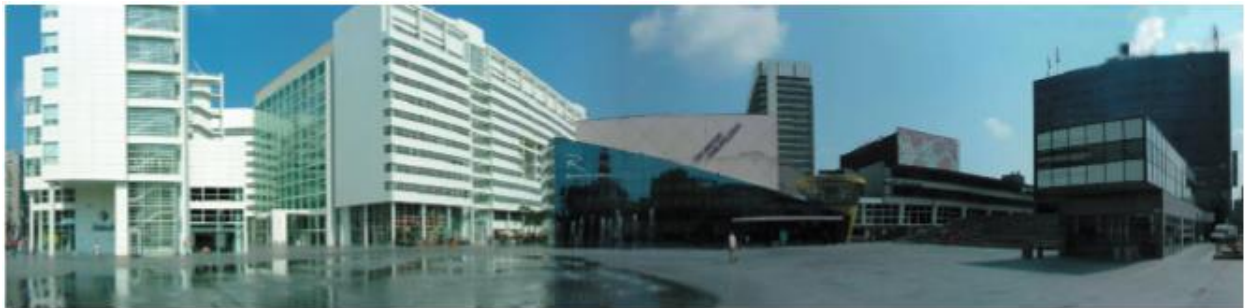
Figure 258. The Hague's Spuiplein with from left to right City Hall by Meier Architects (1995), the Anton Philipszaal by Van Mourik and Vermeulen architects (1987), the Nederlands Danstheater by Rem Koolhaas (1987) and the Hotel Central by Carel Weeber (1985). 1080
