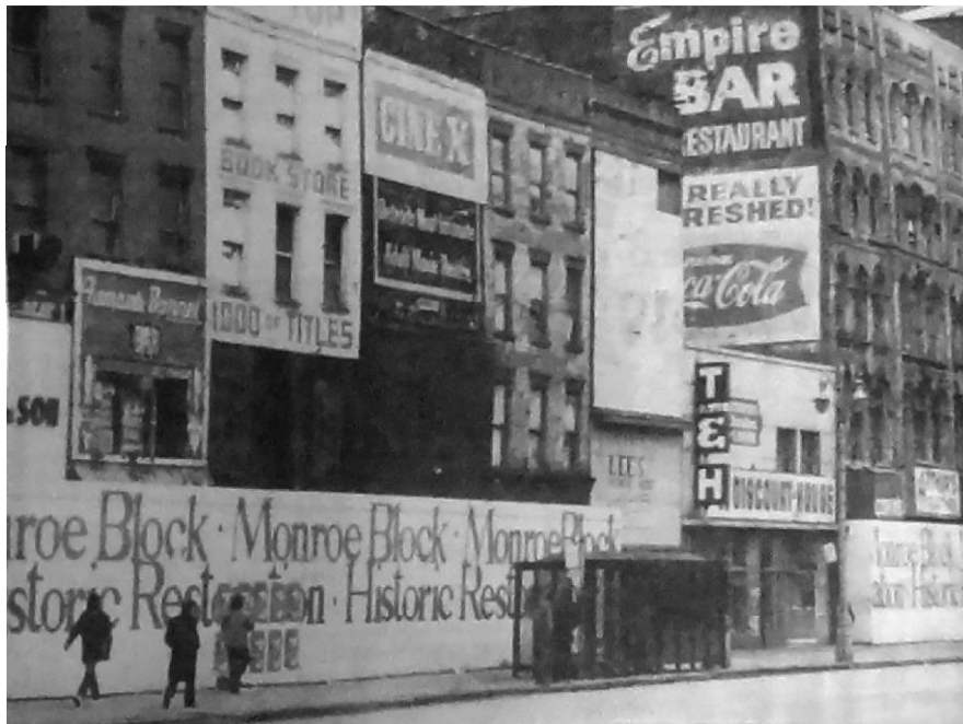
Figure 112. Decay on Monroe Street, promising “historic restoration”. 650
