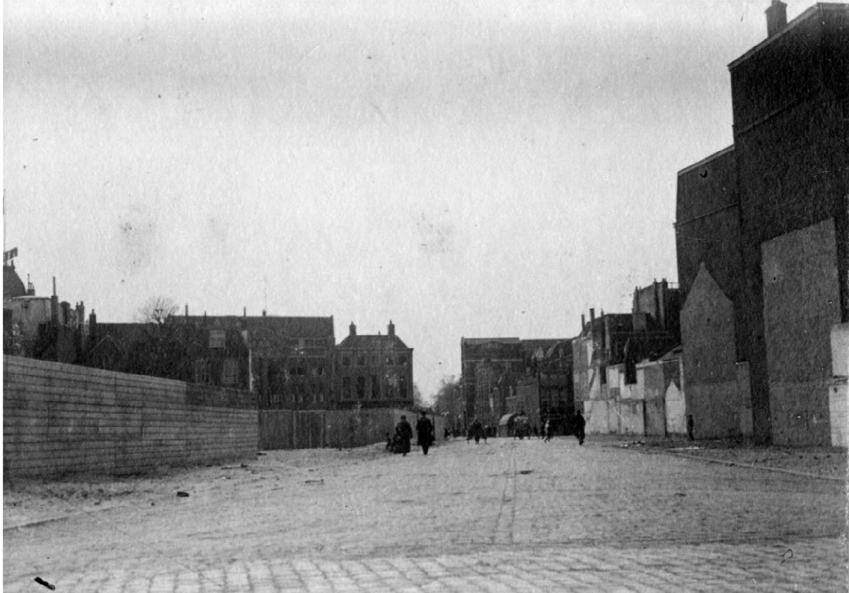
Figure 137. Construction of the Grote Marktstraat, around 1920. 776
