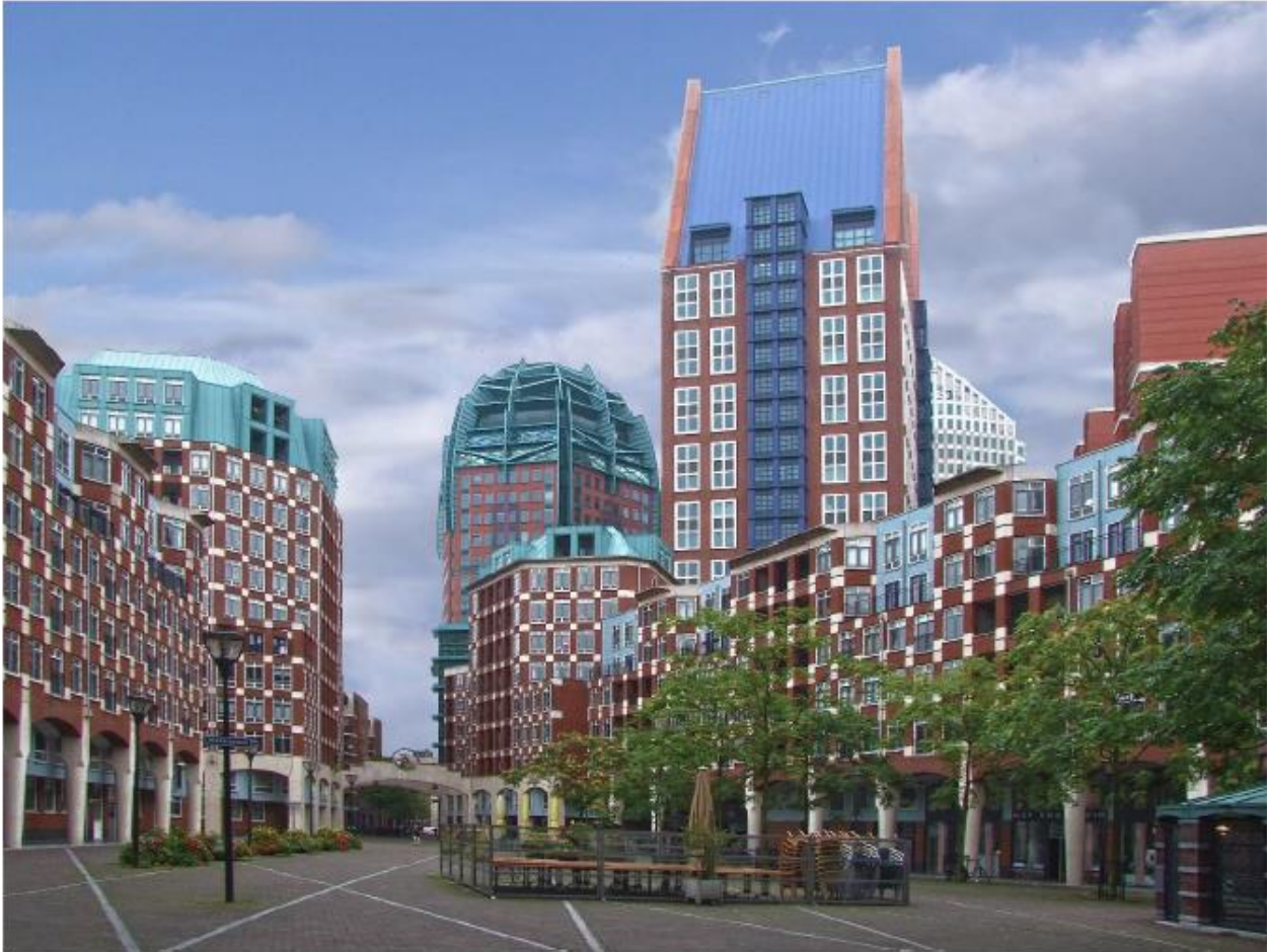
Figure 259. Central Muzenplein square in De Resident, with taller structures embedded into a midrise urban tissue which addresses the street. 1083
