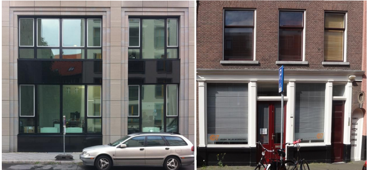
Figure 341. Transparent office ground floor on Neue Grünstrasse in Berlin (left), storefront turned into an office with shutters in The Hague (right). 1304
