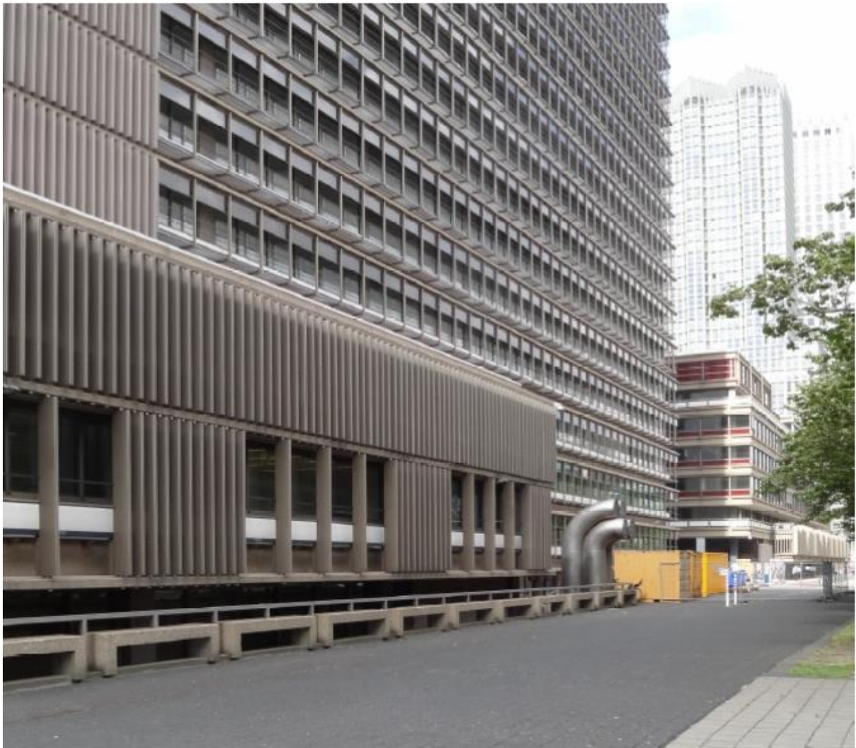
Figure 257. The ministries of Justice and Internal Affairs at eye level: a protective mound, inactive ground floor and ventilation shafts for a subterranean nuclear bunker. 1071
