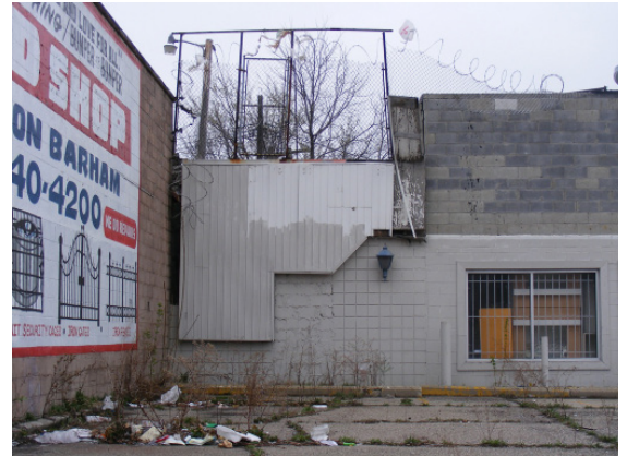
Figure 9.4 High priority code violation
