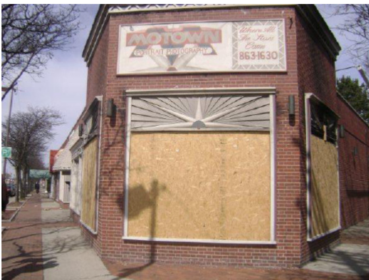
Figure 4.1. Secured vacant building on Livernois Avenue
