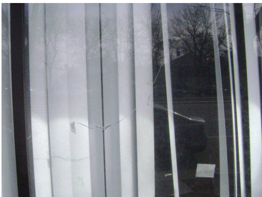
Figure 8.9. Broken window on the 19400 block of Livernois
