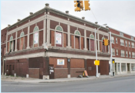
Figure 7.7 Odd Fellows Hall before renovation
