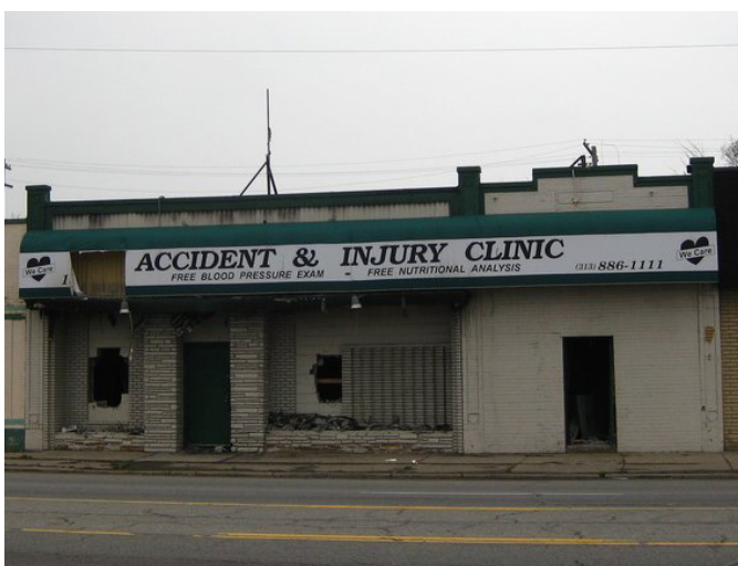
Figure 9.6 Open and unsecured building
