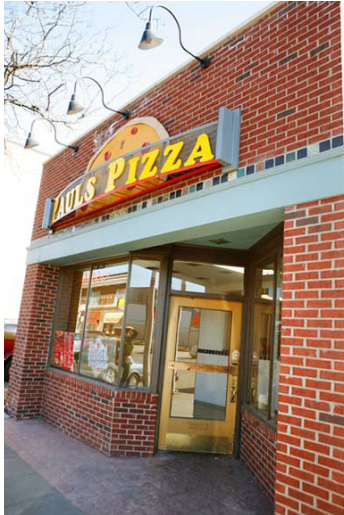
Figure 3.5 An improved facade thanks to Refresh Detroit
