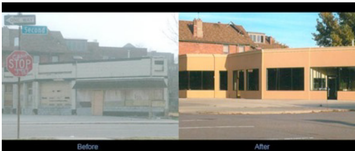
Figure 10.2: A successful reinvestment due to the NAP, 3574 Second Avenue in Detroit
