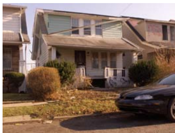
Figure 2.13. Residential Conditions: Example of “Needs Improvement”
