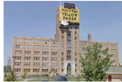
Figure 6.12 Bell Building Source: Google Maps, imagery date 2007
