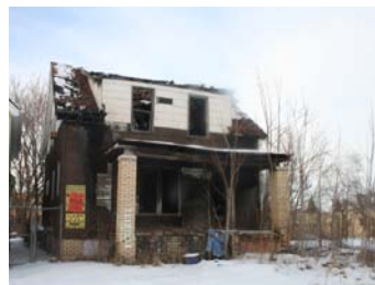
Figure 2.14. Residential Conditions: Example of “Candidate for Demolition”
