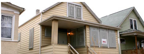
Figure 4.7: House Secured Using the VPS System
