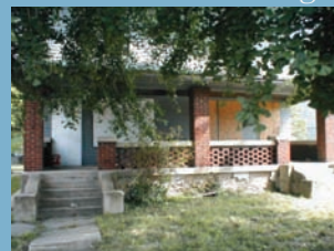
Figure 4.4: East Third Street Before Painting
