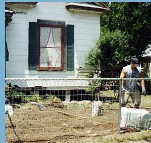
Figure 4.3: Painted Boards on Southside Preservation Hall
