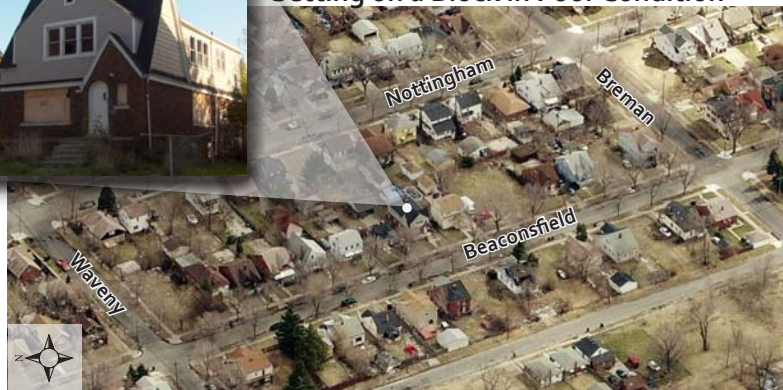
Figure 7.13: 4158 Beaconsfield in its Setting on a Block in Poor Condition
