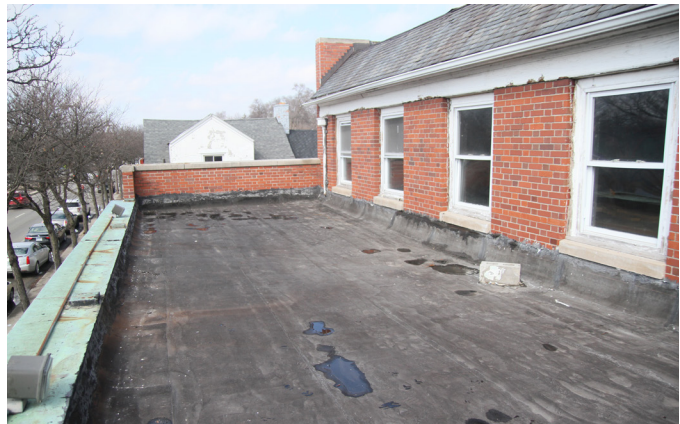
Fig. 37: Existing second-floor roof space
