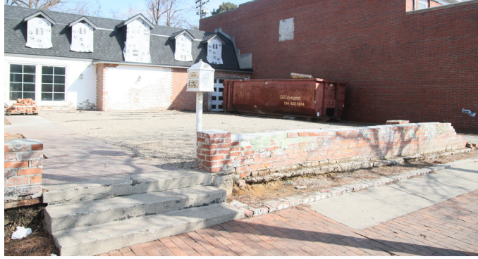
Fig. 38: Stairs to courtyard above sidewalk grade
