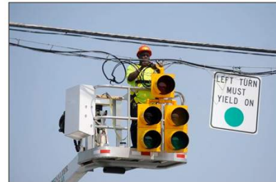
A worker attempts to repair a traffic light during a power outage after a severe storm.
