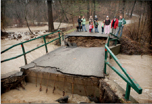
Residents of a Grand Rapids neighborhood look at a bridge washed away in April of 2013. The bridge was what connected residents from the neighborhood to main roads.
