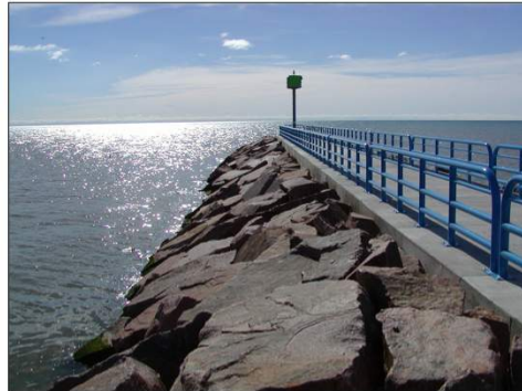
Breakwater in Michigan made from salvaged materials.
