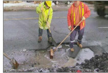
Road crews in Toronto attempt to clean up cracked pavement in January 2014
