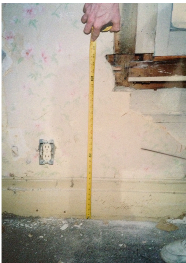
Figure 15: P11 determined that the house used to have taller molding after carefully examining the unpainted area after he removed the first layer of the drywall.
