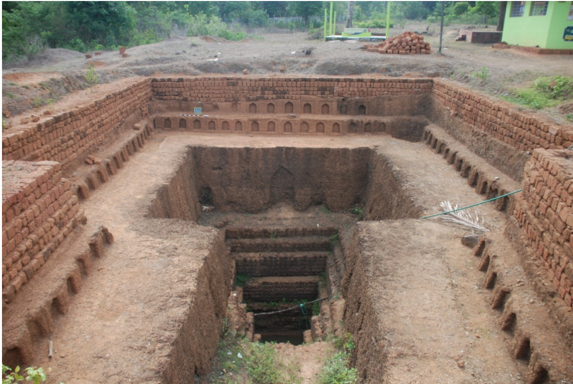
Figure 5.85: Tank, Complex Shape with arched niches, Ikkeri (KIN 188)
