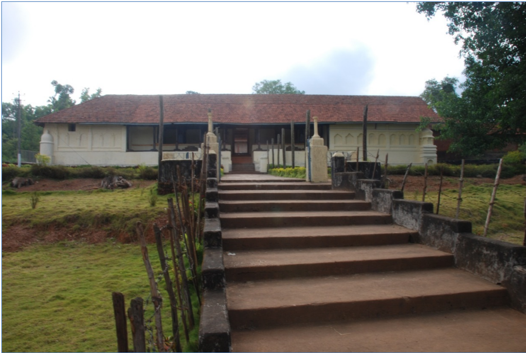
Figure 5.18: Rameshwara Temple Complex, Keladi, exterior (KIN 2)
