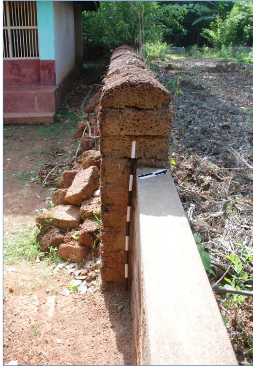
Figure 5.35: Laterite Temple Wall, cross-section, Keladi (KIN 238)
