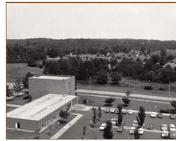
The site of the future Bentley Historical Library.
