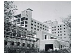
South Quad Dorm under construction, May 1952
