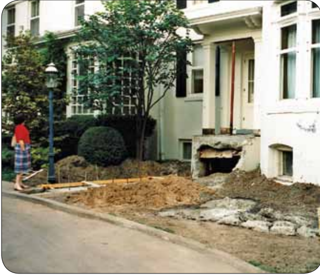
Preparations for a handicap ramp
