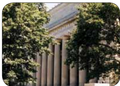
Angell Hall Renovation
