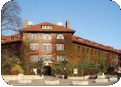
West Engineering Building
