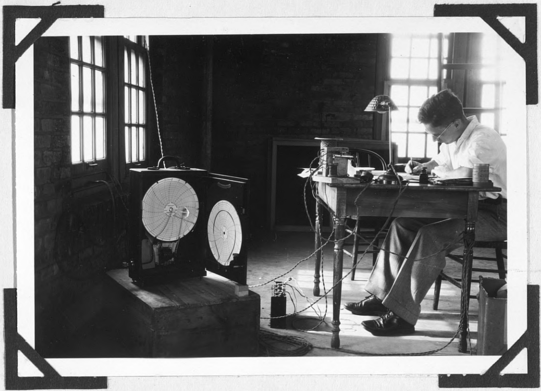
Control Station in the Union Tower Room. Gauge Connected to the Window at the Left.
