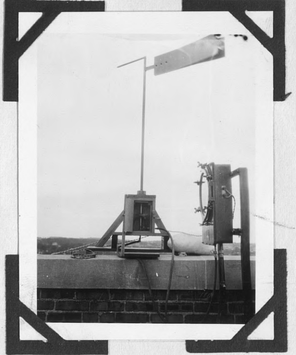
Direction Control on Vane.
