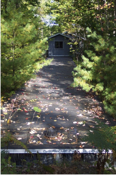
Fig. 10. A view along the roof of the underground laboratory space of the UMBS Soil Biotron, a belowground laboratory that provides rare opportunities to view and study roots, fungal hyphae, soil invertebrates, and microbes in situ in the upper 1.2 m of soil.
