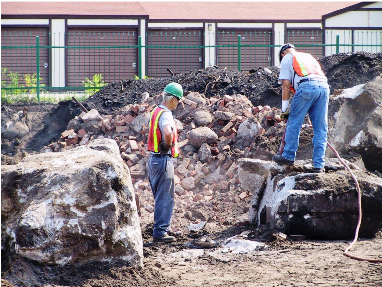
Figure 8.4: Workers removing concrete, asphalt, and bricks (photo credit: KNC)
