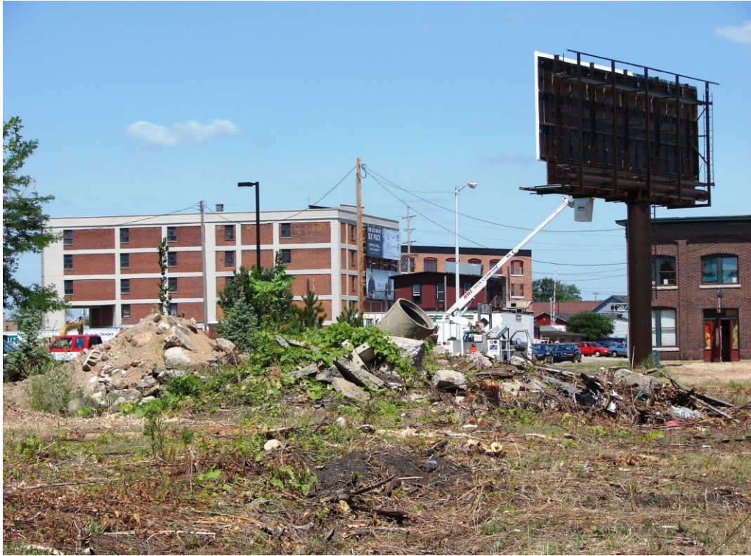
Figure 8.2: Industrial debris on the site before clean-up efforts (photo credit: KNC)
