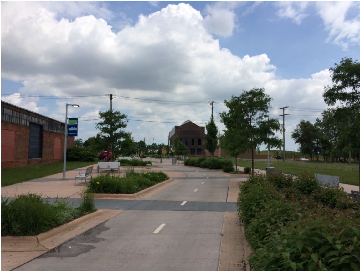
FIGURE 20: THE AT-GRADE PORTION OF THE DEQUINDRE CUT NEAR THE DETROIT RIVERFRONT. PHOTOGRAPH BY AUTHOR 2013.
