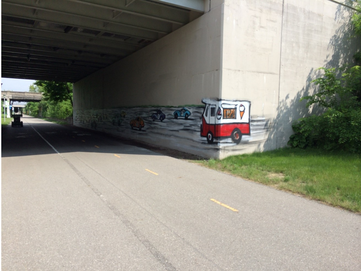
FIGURE 23: CURATED GRAFFITI ON THE DEQUINDRE CUT. PHOTOGRAPH BY AUTHOR 2012.
