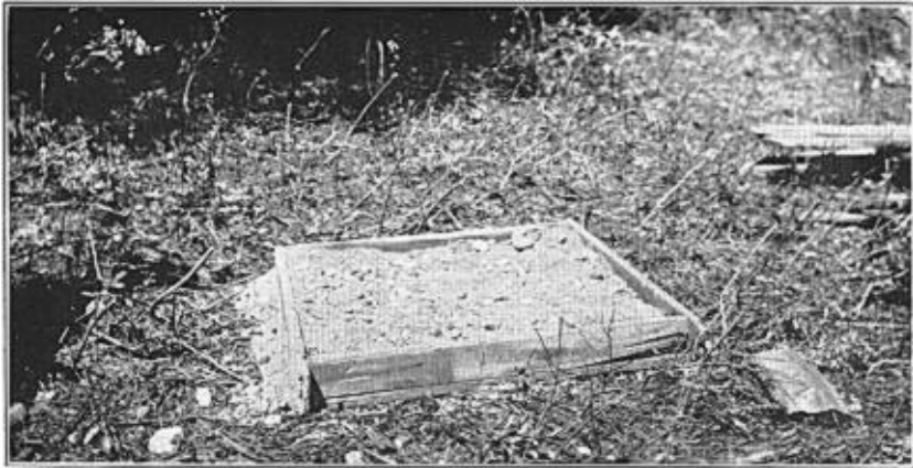
5. Box of old boards filled with gravel. Used where bottom is soft.
