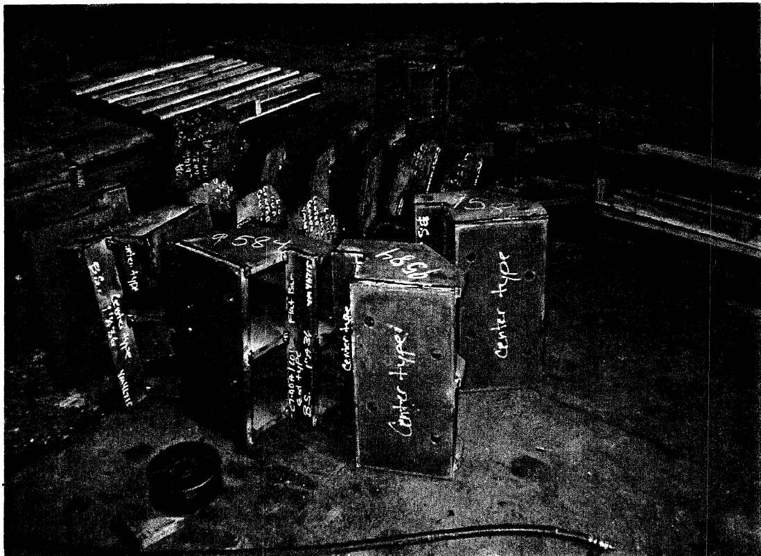
Photo 30. Finish welded dogging plates.
