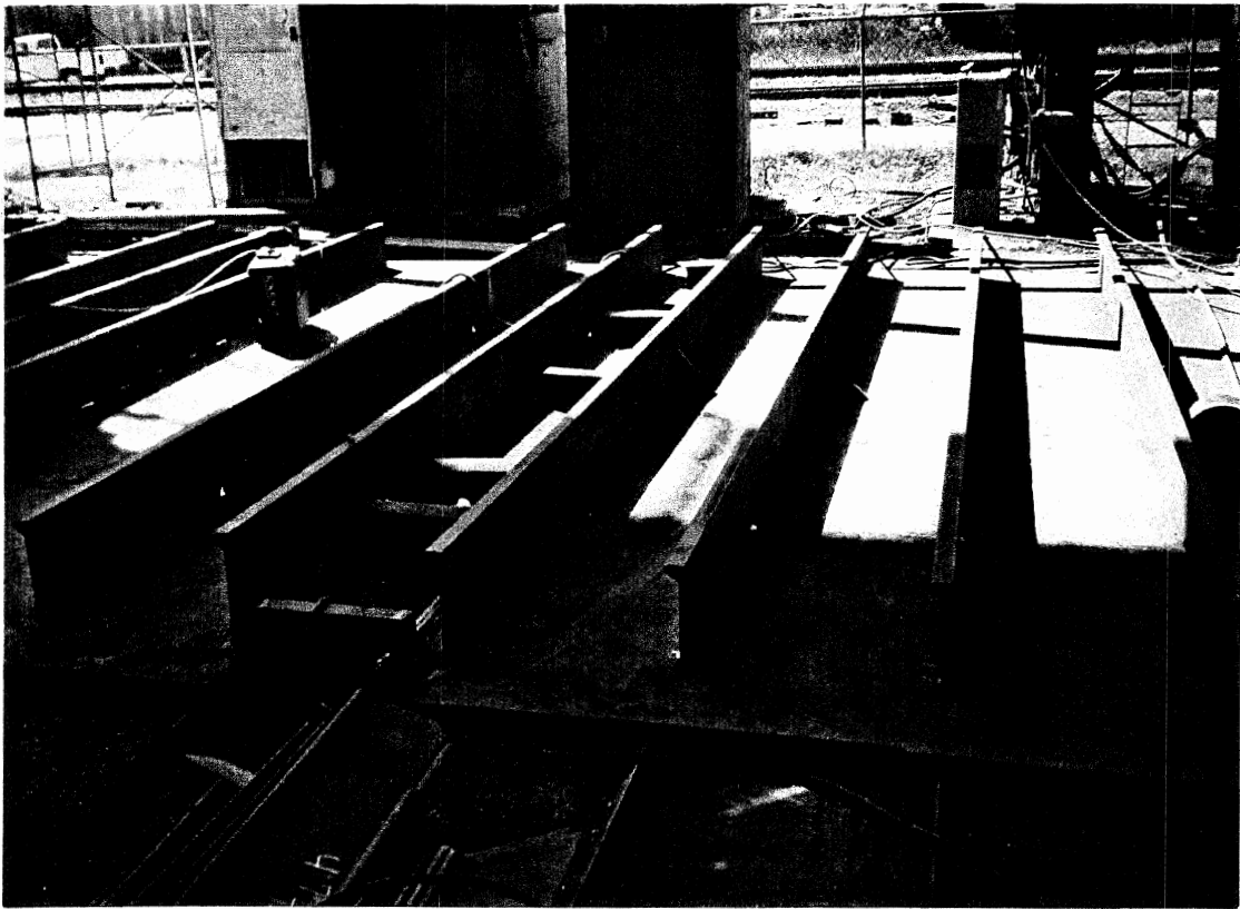
Photo 2. Welded temporary supports of scrap metal.
