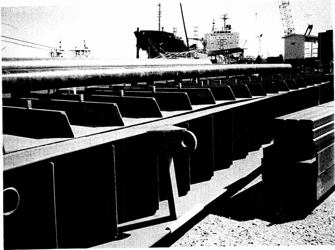
Photo 1. Welded pad eye with added angle support and chafing guard around bottom plate.
