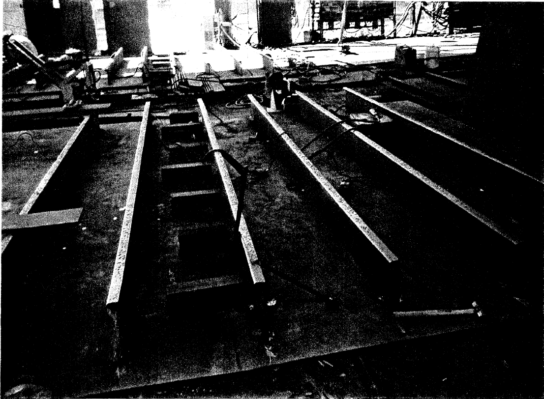
Photo 3. Welded butt joint strongbacks.
