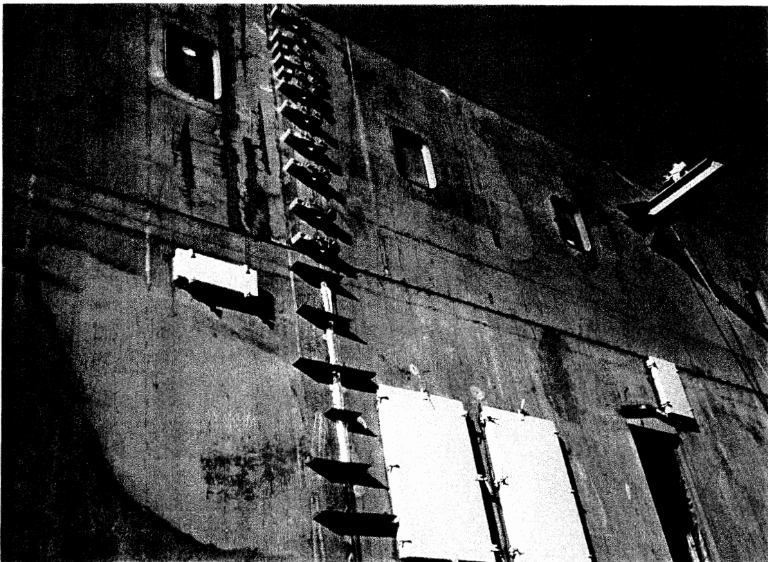
Photo 12. Deckhouse erection butt joint - shows the old method (file welded flat bar strong backs) and a new method (stud-welded threads with boxed strong backs) of alignment.
