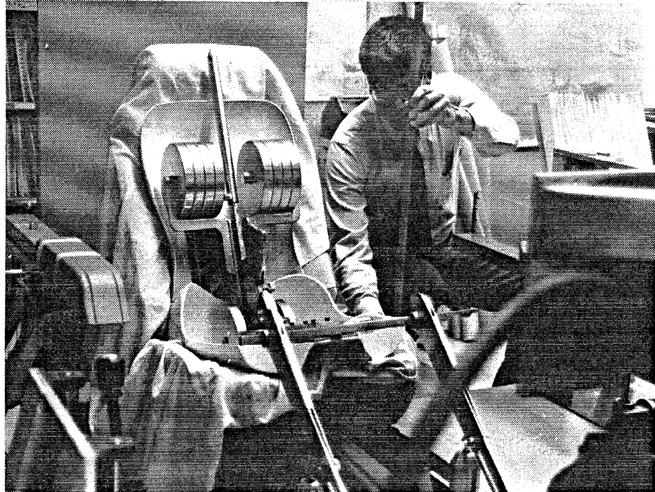
Figure 7. H-point calibration of seating buck.
