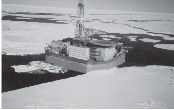
Figure 1.1: Photograph of the Molikpaq in the Canadian Beaufort Sea covered with ice (Timco and Johnston, 2003)
