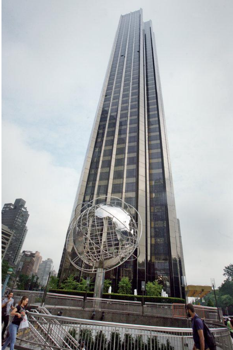
Figure 1.1 Trump International Hotel & Tower at 1 Central Park West, façade by Philip Johnson. The architect did not remove the old façade but instead overlaid a bronze-colored glass set in a grid of dark anodized aluminum. (Vivian Marino, “$33 Million Penthouse on Central Park West,” New York Times , February 1, 2015.)
