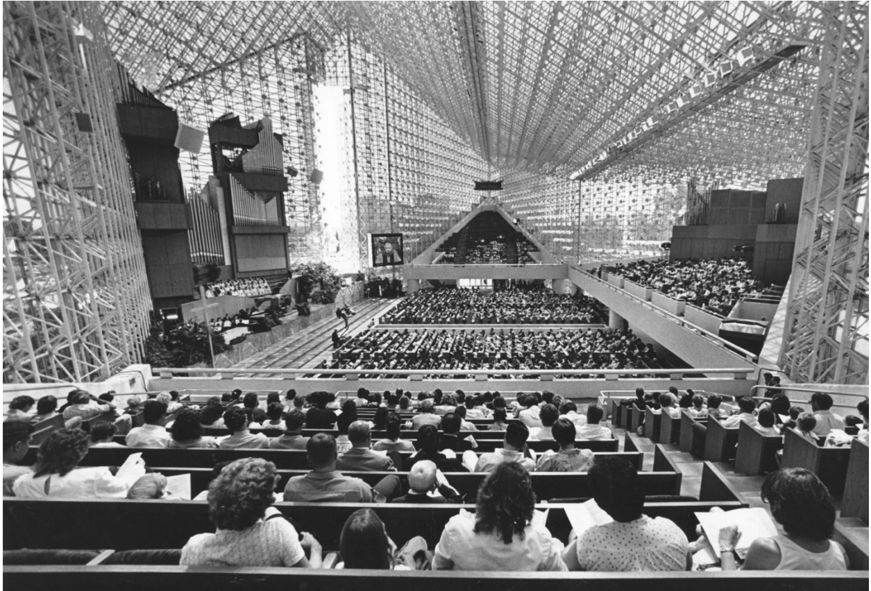
Figure 5.37 Interior view from upper-level seating, Crystal Cathedral, Philip Johnson, Garden Grove, California, 1980. From here all of the elements of the church are visible: enveloping glass structure, concrete piers, entry fountain, stage, organ, televisual equipment, jumbotron, and open eighty-foot doors.
