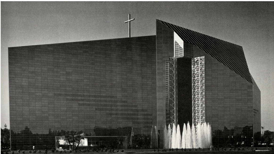
Figure 5.20 Exterior view, Crystal Cathedral, Philip Johnson, Garden Grove, California, 1980. Eighty-foot mechanical doors shown open and fountain jets on. Both features are outsized versions of key design elements from the Garden Grove Community Church but no longer connect walk-in and drive-in worshippers.
