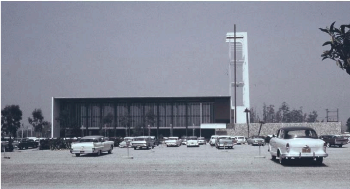
Figure 5.17 Exterior view showing drive-in arrangement, Garden Grove Community Church, Richard Neutra, 1962.
