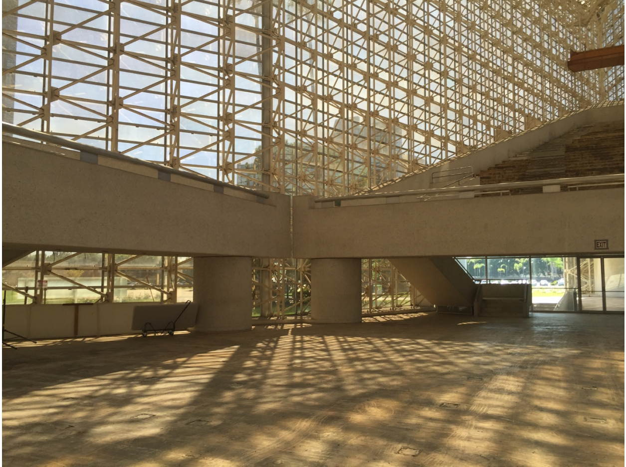
Figure 5.32 Interior view looking back at concrete piers, Crystal Cathedral, Philip Johnson, Garden Grove, California, 1980. Showing the horizontal datum within the main space of the church. (Photograph by author)
