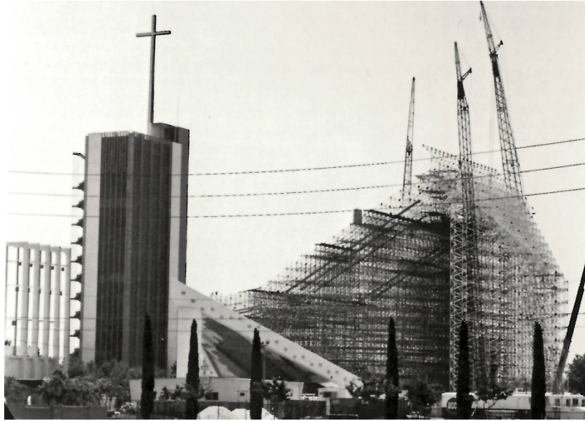
Figure 5.5 Construction photograph, Crystal Cathedral, Philip Johnson, Garden Grove, California, 1980.
