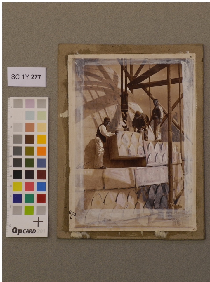
Figure 3.32 Photographs of workers on the construction site of the church. Bottom image shows photograph being used as a base and enhanced with a color wash, possibly in preparation for use in publication. (Archives historiques du diocèse de Paris)
