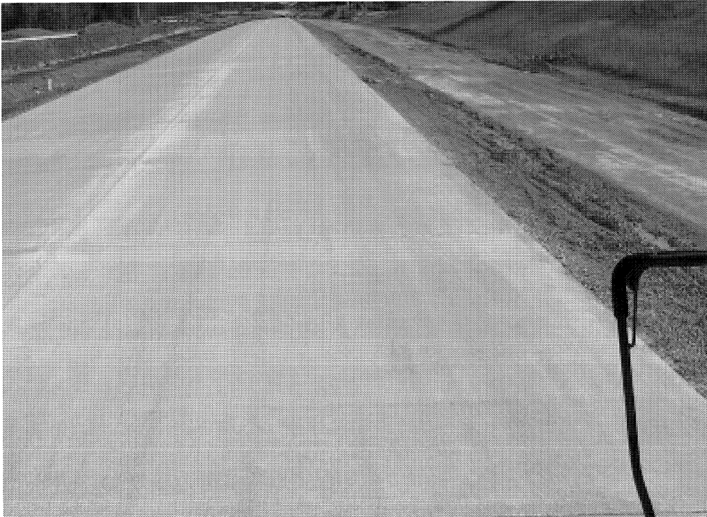
Site 4 (Novi) Long View, Looking Downstream.
