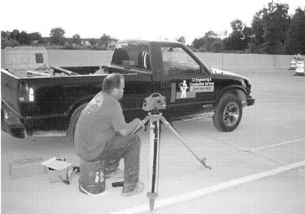
Optical Level at Site 2
