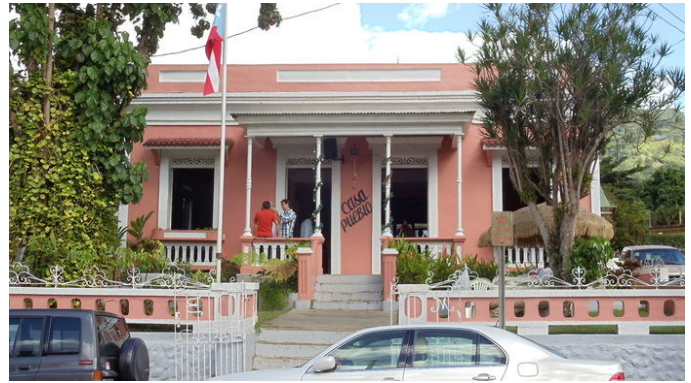
(Right) Casa Pueblo Main Building
