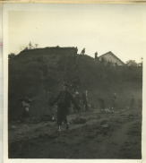
The way the R.R. is being built. All by man power. Tons of dirt carried on men's shoulders. Taken at sunset.
