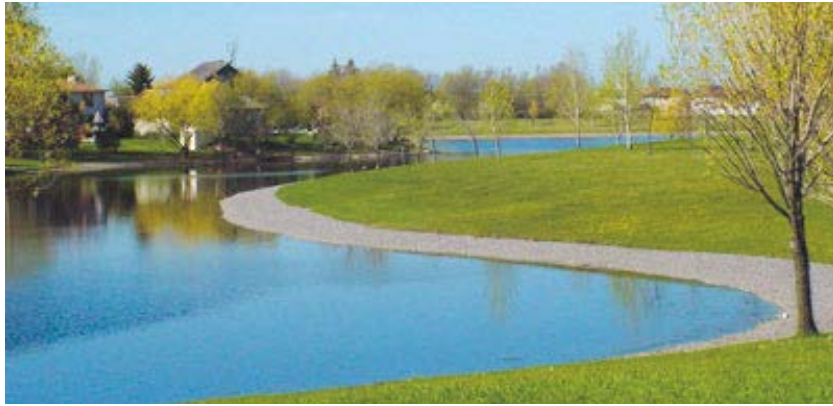
Figure 9. Artificial retention basin creating an urban landscape feature while storing stormwater runoff (Retention Ponds, 2020).
