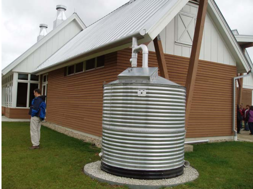
Figure 10. Above ground cistern collecting rainwater from the roof of attached structure (Rainwater Harvesting & Cisterns, n.d.).
