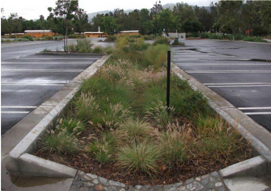
Figure 8. Bioswales collect stormwater off of adjacent parking lots (Gibb, 2015).
