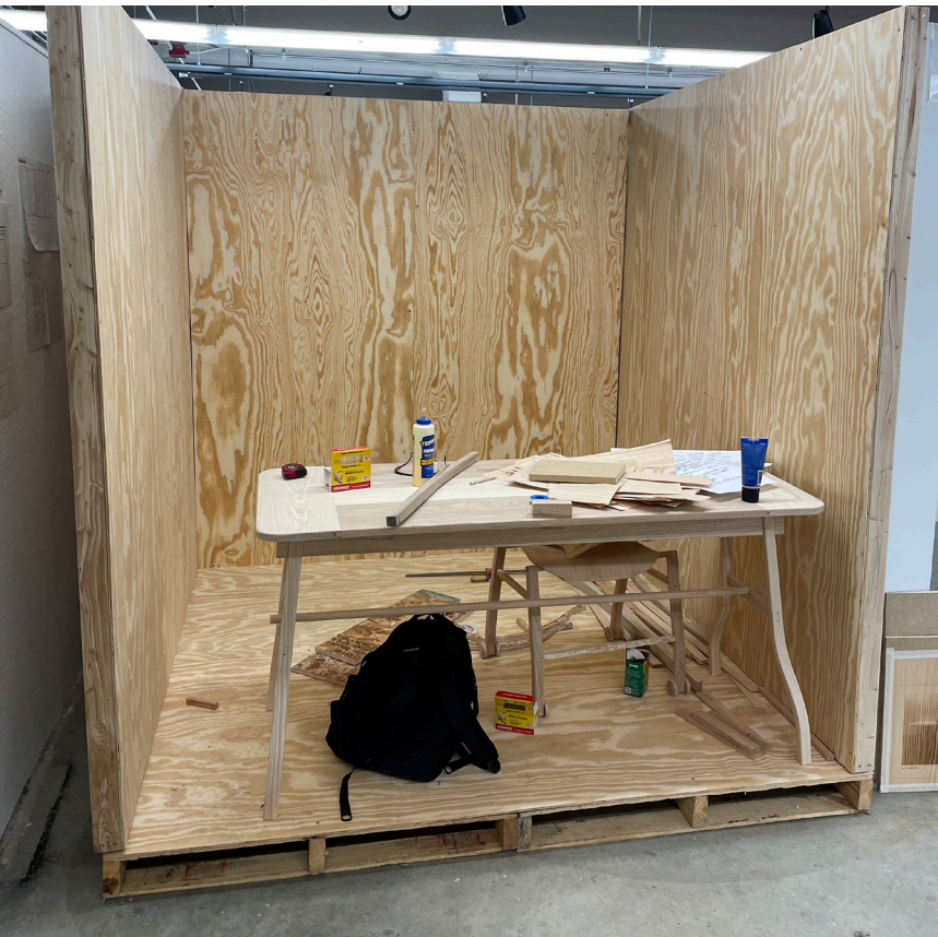
30 FLOOR &amp; WALLS ERECTED IN THE EXHIBITION SPACE
