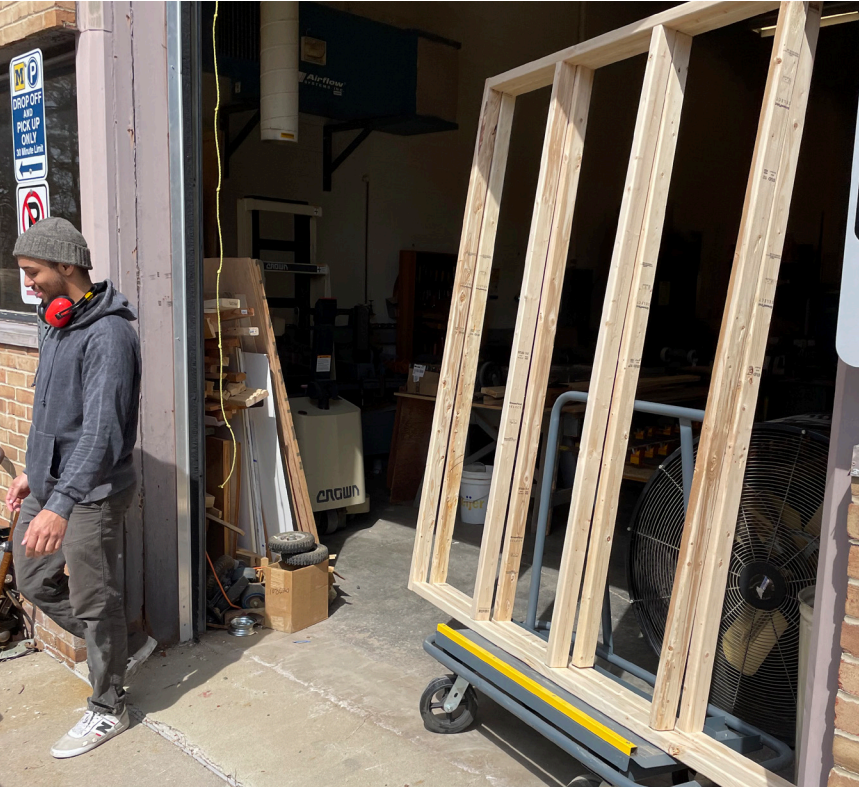
29 FRAMES BEFORE BEING COVERED WITH PLYWOOD
