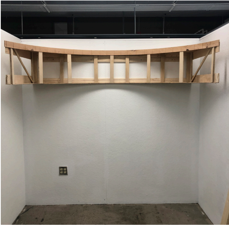
Wooden frame attached to wall.
