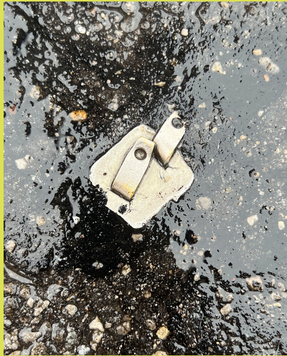
A phone charger stuck in the cement
