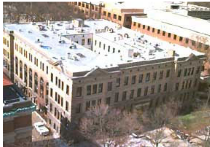
Figure 12: S.T. Dana Building – Pre construction
