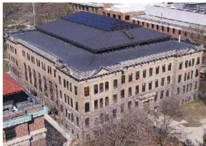
Figure 13: S.T. Dana Building – April 2001
