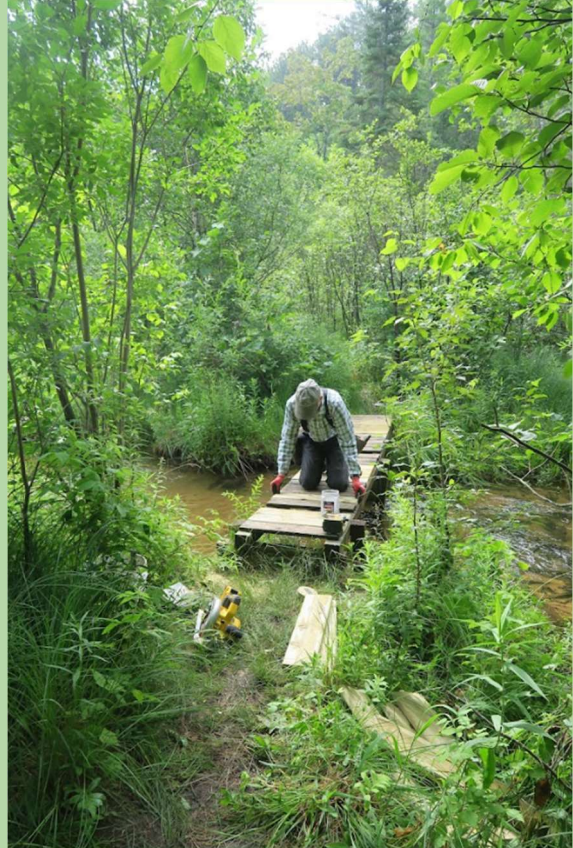
Image 9. Steward Repairs Gorge Bridge; Sara Thiessen 2023
