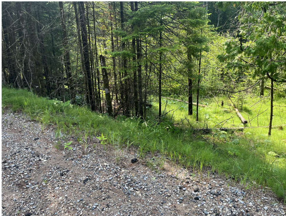
South edge of Hogsback Road just East of Carp Creek
