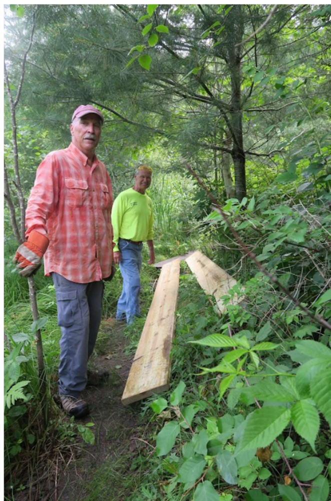
Image 8. Bug Camp Stewards Repair Gorge Trail Bridge; Sara Thiessen 2023
