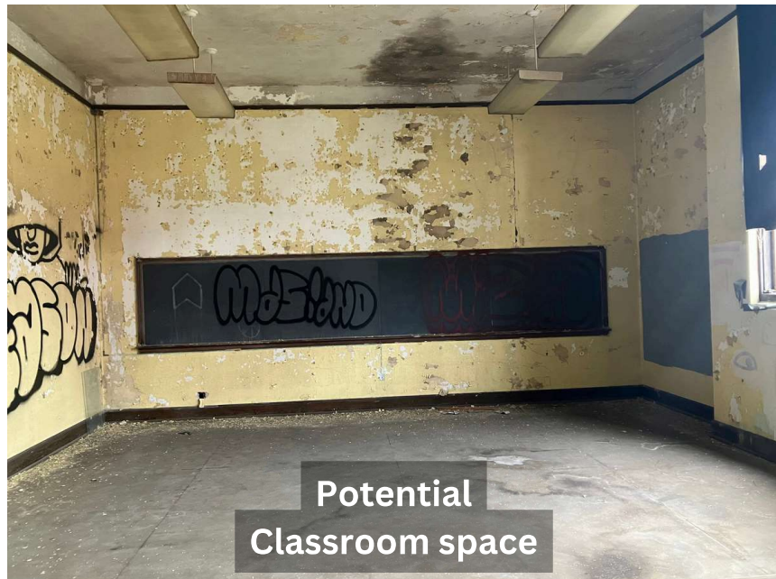
classroom space on 2nd floor
