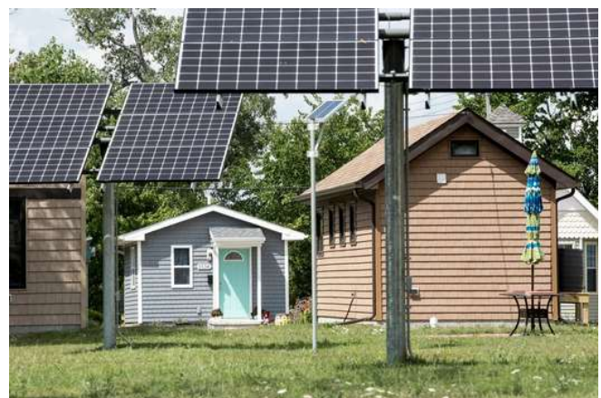
Figure 67. CCSS Tiny Homes in Detroit w/ ground-mounted solar panels to supply energy. Each Tiny Home has a 1.8 kW solar array [8].
