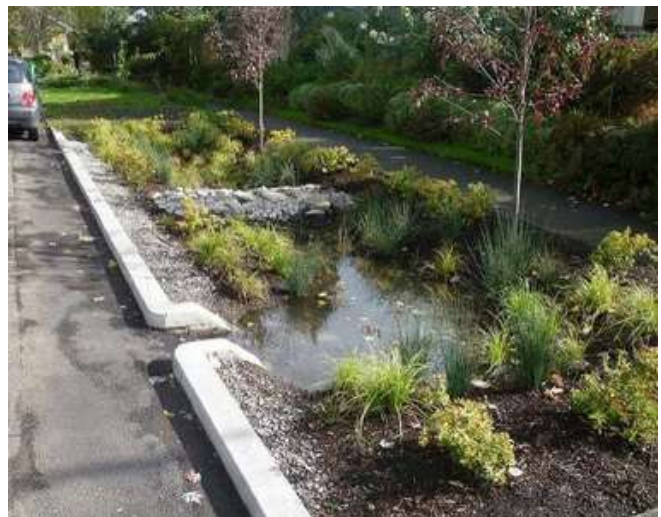
Figure 63. Curbside bioswales after a rainstorm. [80].
