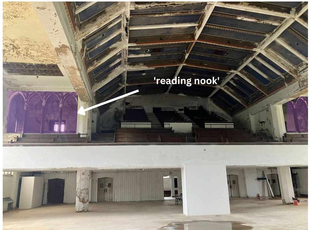
View of atrium looking toward entrance
