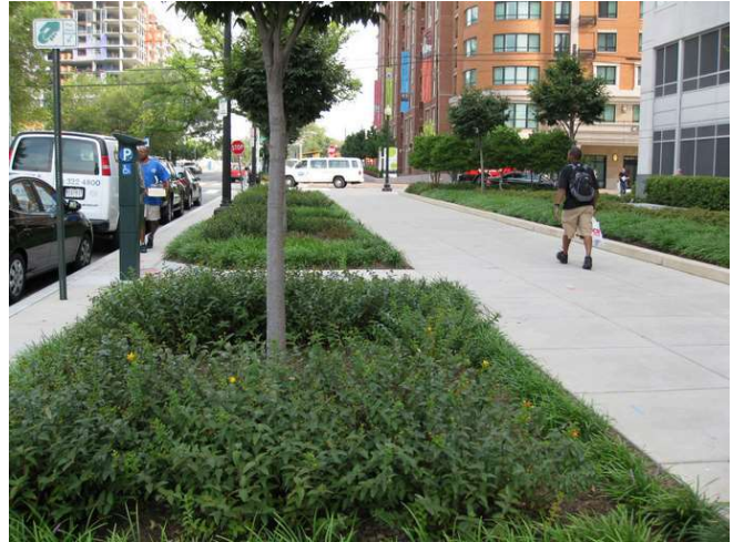
Figure 62. Curbside bioswales during dry weather [79].
