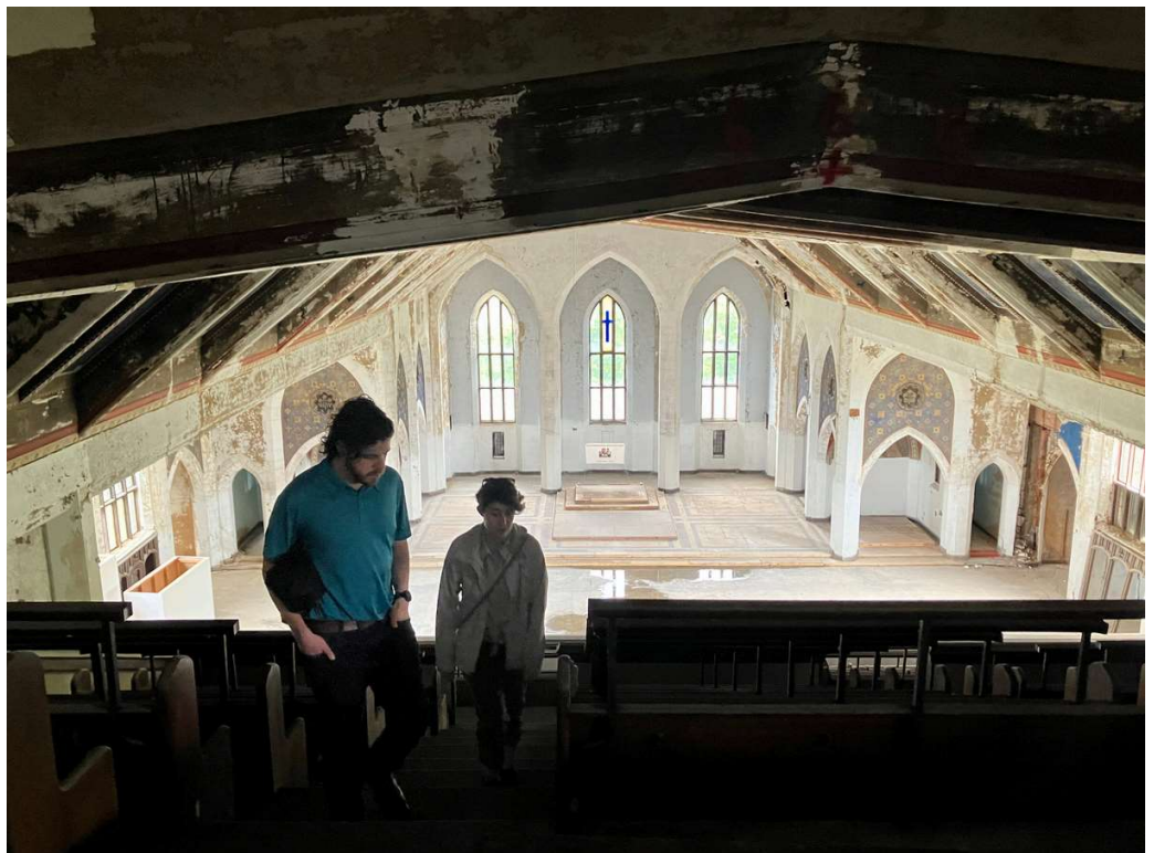
View of atrium from riser seating
