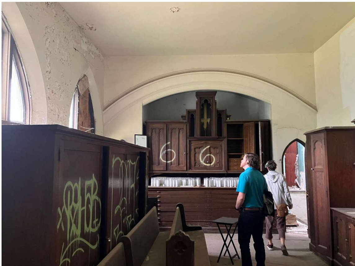
Left of pulpit side room looking toward doorway to pulpit
