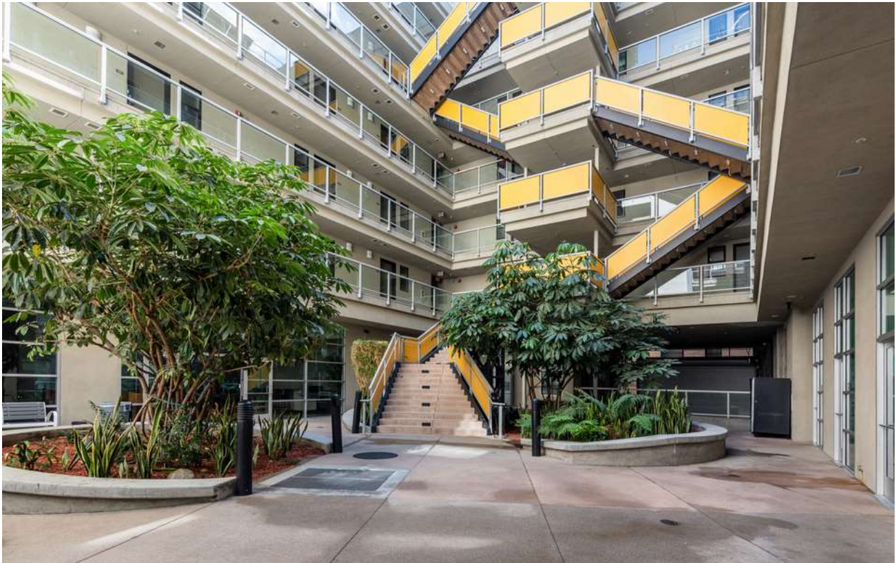
The central atrium at New Genesis, showing its open corridors and abundance of natural light. Design Resources for Homelessness
