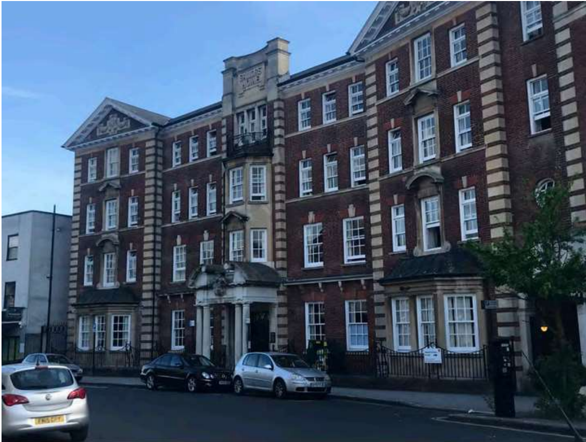
The Booth Centre from the street entrance side. Design Resources for Homelessness
