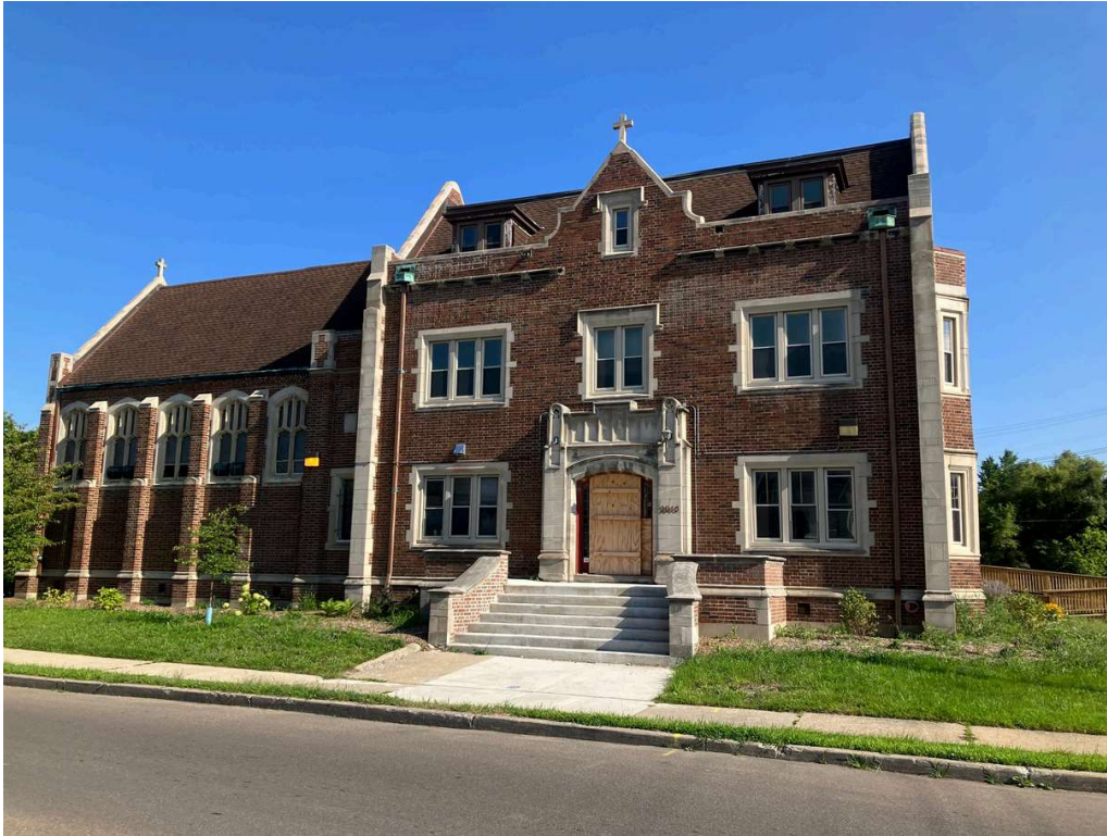
View of Webb Side of Building
