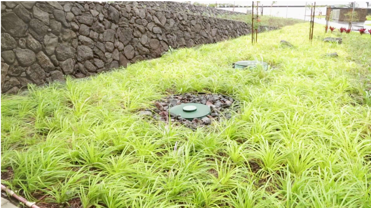
Photo 9. Storage Tank Access. Source: Storage Tank Access. University of Hawai'i Sea Grant. (2019). Water Reuse – Hawai'i Sea Grant . Hawai'i Sea Grant. Retrieved March 26, 2024, from https://seagrant.soest.hawaii.edu/water-reuse/
