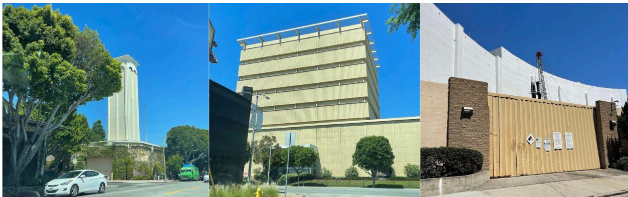
Figure 1. First image Packard Well Site, middle West Pico Drill Site and last photo of the Beverly Center.
