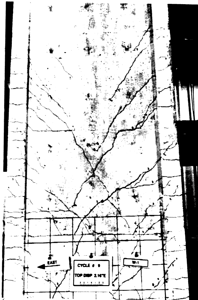
Fig. 4.4 : Formation of Compression Struts in the Top Portion of W-1 during Cycle 9.
