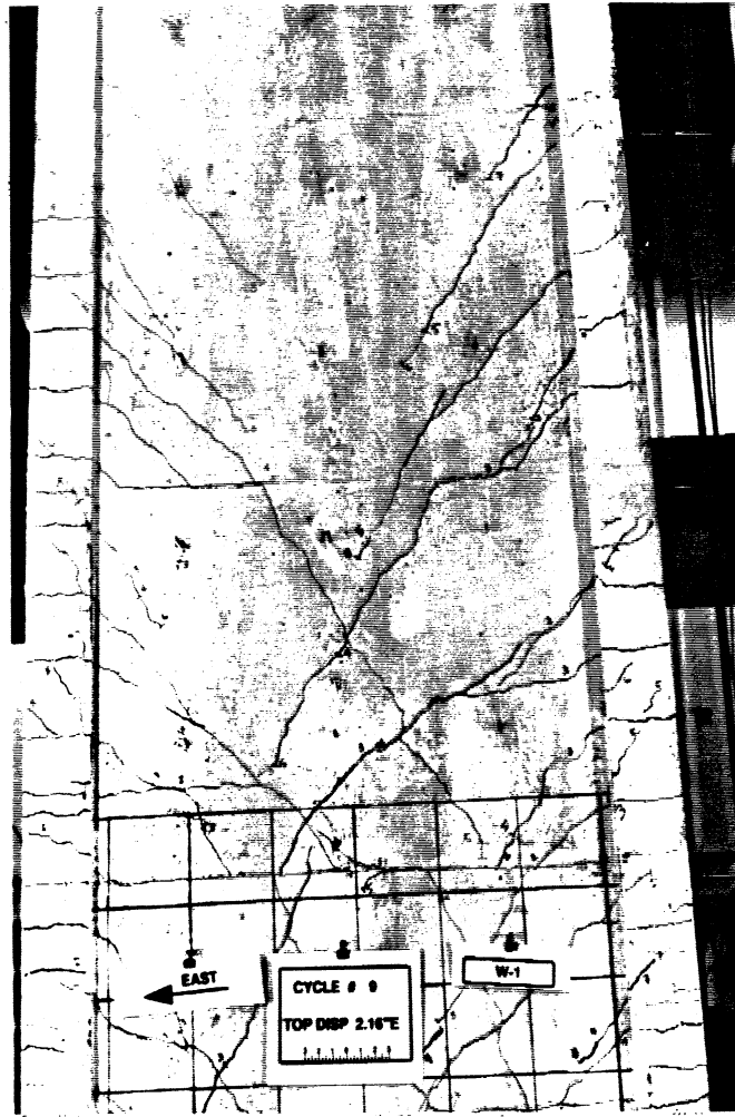
Fig. 4.4 : Formation of Compression Struts in the Top Portion of W-1 during Cycl
