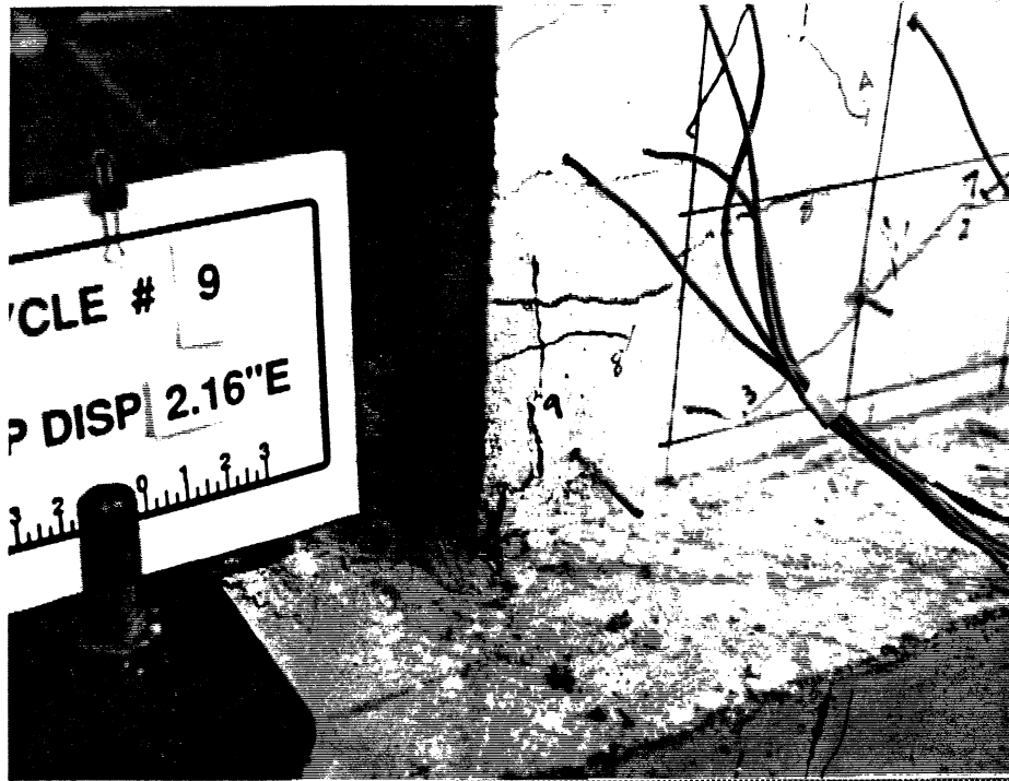
Fig. 4.5 : Initiation of Crushing in East Boundary Column of W-1 during Cycle 9.
