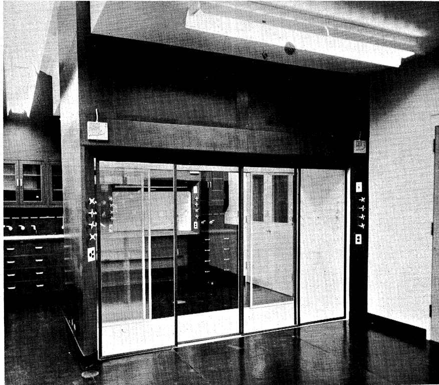
Figure 2.13 Photograph of a "walk-in" hood capable of housing assemblies 6-1/2 feet high. A standard chemistry hood-bench assembly is visible in the background (5)
