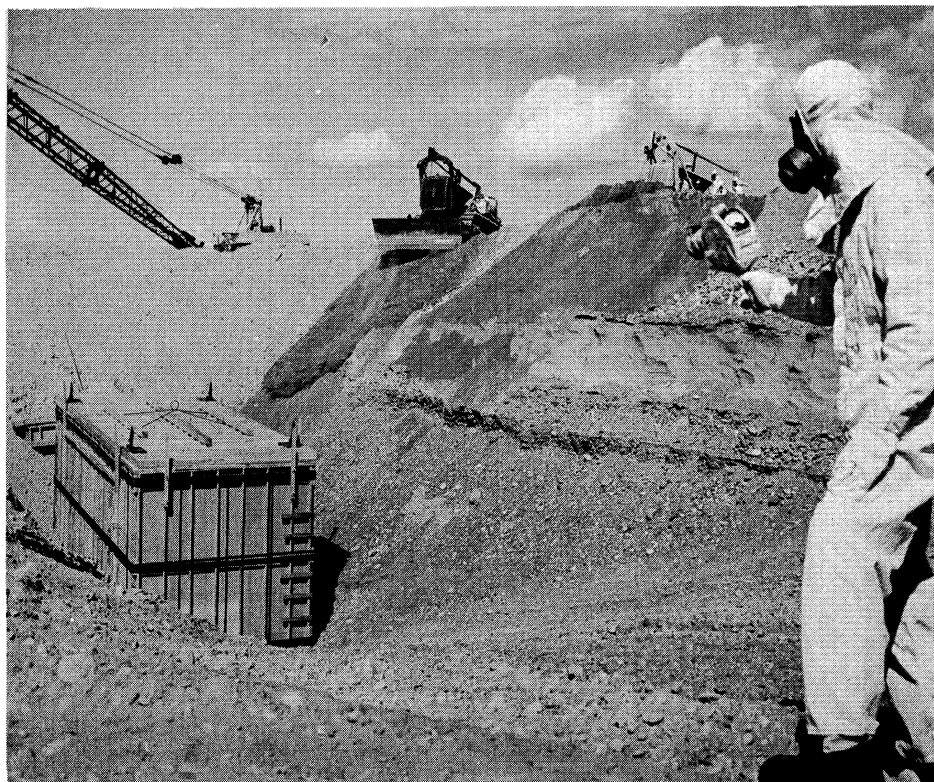
Figure 1.9 Burial of highly radioactive waste at Hanford (Courtesy of General Electric Co.)
