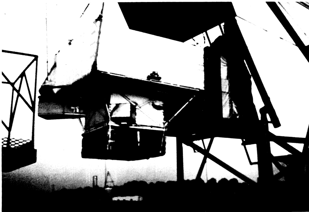
Figure 3. - Gondola on launching truck
