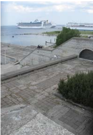
Figures 157a-c Linnahall, built near the passenger ferry terminal in the 1980s, is already in need of significant renovations.
