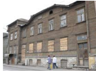
Figure 121 Historic wooden row houses in Põhja-Tallinn were built in the early 1900s.
