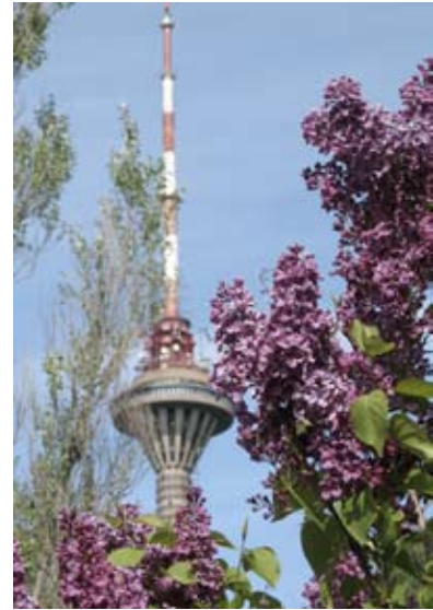
Figure 155 The Teletorn punctuates views from many places in the city, and dominates the skyline of the Botanic Gardens.
