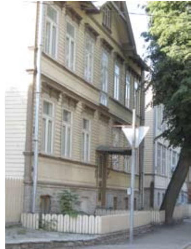
Figures 183b-d Renovated townhouses face abandoned property on Jakobsoni Street.
