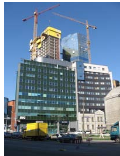
Figures 166a-b Boomtown's new downtown is under construction in glass.
