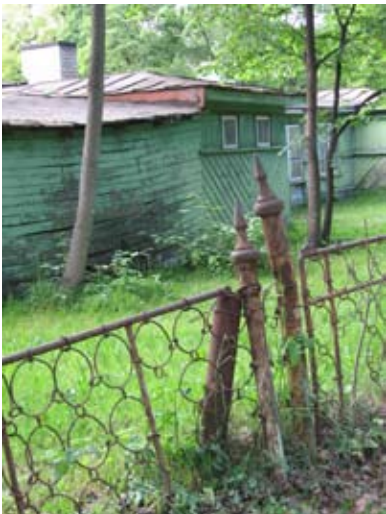
Figure 62 A few outlying buildings on the Kadriorg grounds have fallen into disrepair.
